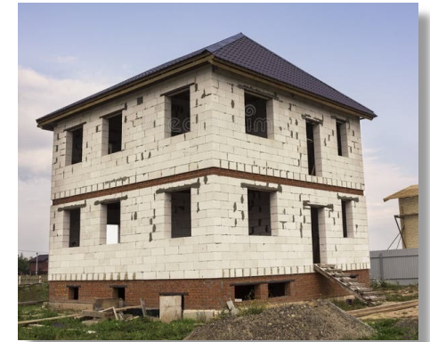
Concrete bricks masonry
