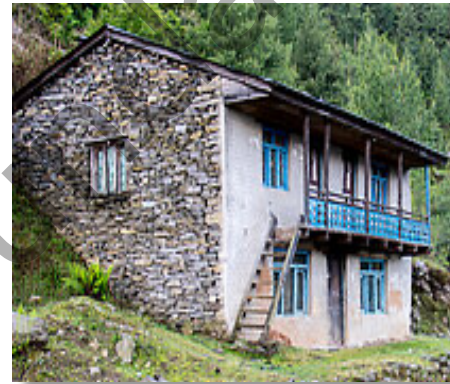
Rubble stone masonry
