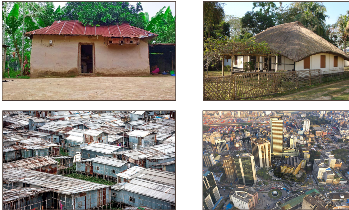
Figure 7-1. Different construction types in Bangladesh Top-left: Adobe / earthen house; Top-right: Bamboo house with thatched roof; Bottom-left: C.I. sheet slum dwellings in Dhaka; Bottom-right: High-rise reinforced concrete structures in Dhaka
