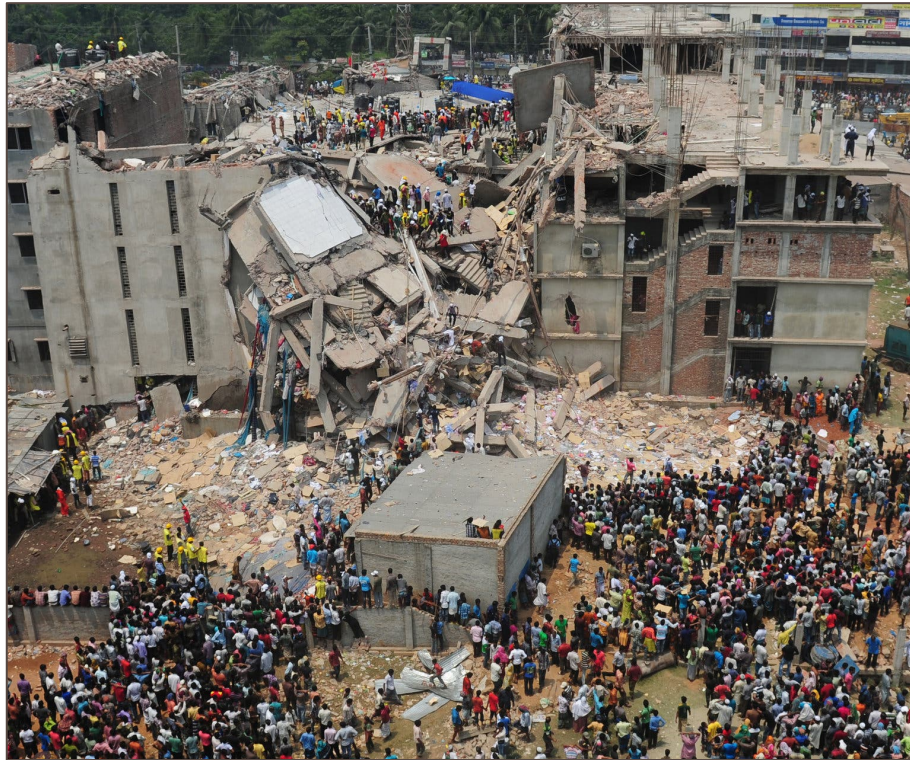
Figure 1-3. Collapse of Rana Plaza on 24 th April 2013.
