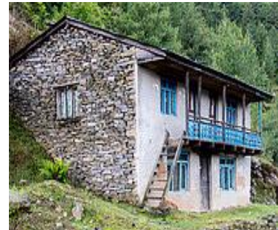
Rubble stone masonry
