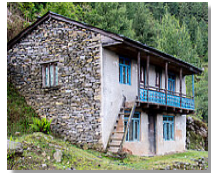
Rubble stone masonry
