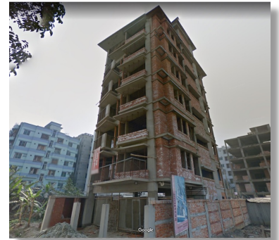
Reinforced concrete buildings
