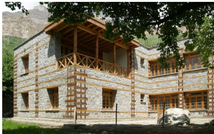
Figure 4.8 Reinforced rubble stone masonry with horizontal timber elements, Pakistan (Photo: T. Schacher)
