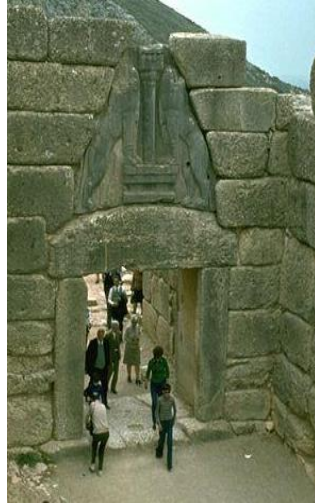
Figure 2.40 Lion Gate at Mycenae, Greece, 13 th C. BCE, illustrating Post and Beam construction with lateral support (Photo: S. Brzev)
