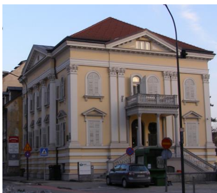
Figure 4.9 A loadbearing brick masonry building, Ljubljana, Slovenia (Photo: S. Brzev)
