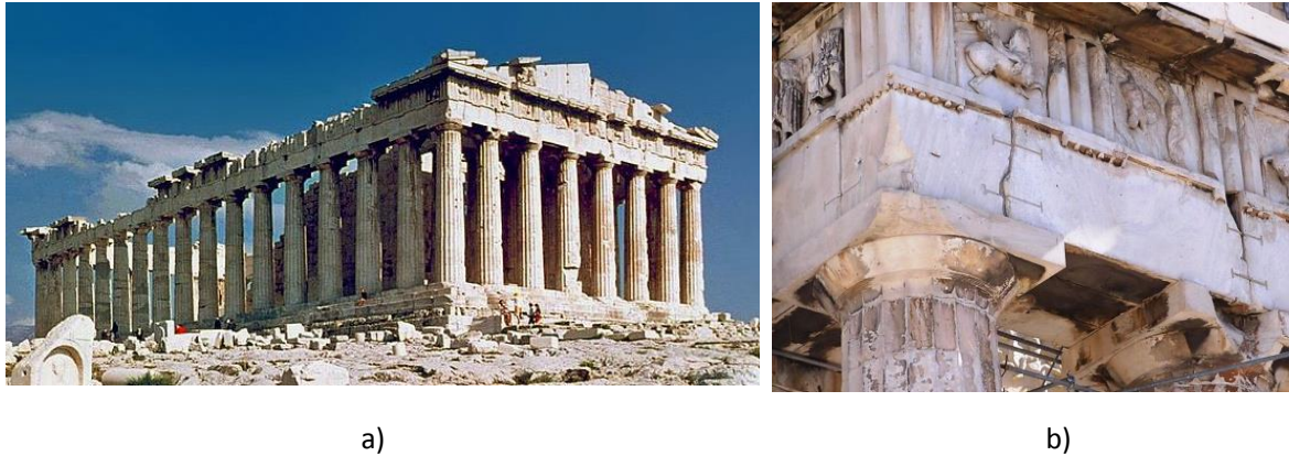
Figure 2.3 Ancient Greek temple Parthenon, Athens, Greece (500 BCE): a) a view of the temple during the structural rehabilitation in 2007, and b) stone columns and beams (lintels) (Photos: B. McEwen)
