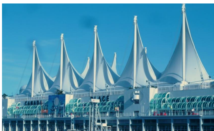
Figure 2.55 Tension fabric roof – Canada Place, Vancouver, Canada (Photo: S. Brzev)
