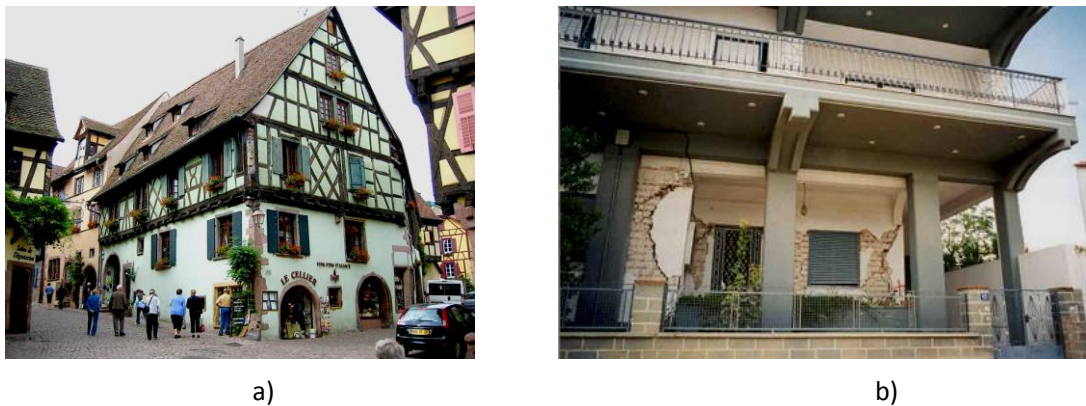
Figure 2.38 Hybrid lateral load-resisting systems: a) stone walls with arches below, wood framing with brick or wattle and daub above in a medieval house, Alsace, France, and b) an old loadbearing brick masonry at the ground floor overlaid by new reinforced concrete frame construction above damaged in the 1999 Athens, Greece earthquake (Photos: a) http://commons.wikimedia.org/wiki/File:Riquewihr_029.jpg ; b) A. Pomonis)
