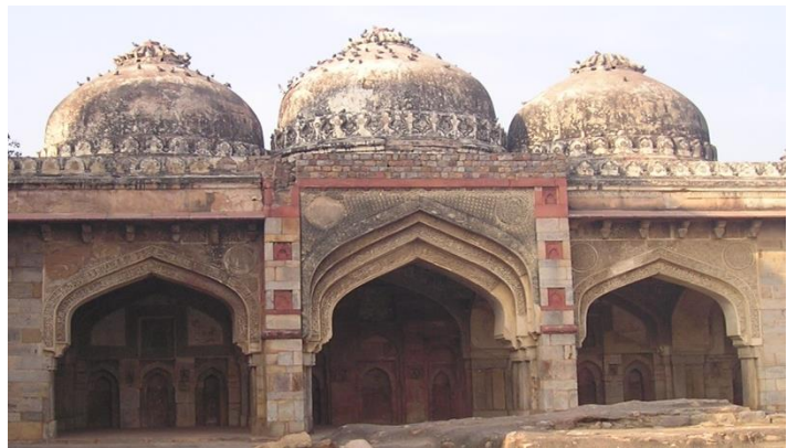
Figure 2.41 Arch structures: a) circular arches in Colosseum, Rome, and b) Arabic arches, Bara Gumbad Mosque, New Delhi, India (Photos: S. Brzev)
