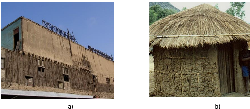
Figure 2.33 Composite wood and earthen construction: a) Quincha construction, Peru, and b) Yamata construction, Malawi (Photos: a) S. Brzev and b) Ngoma and Sassu)
