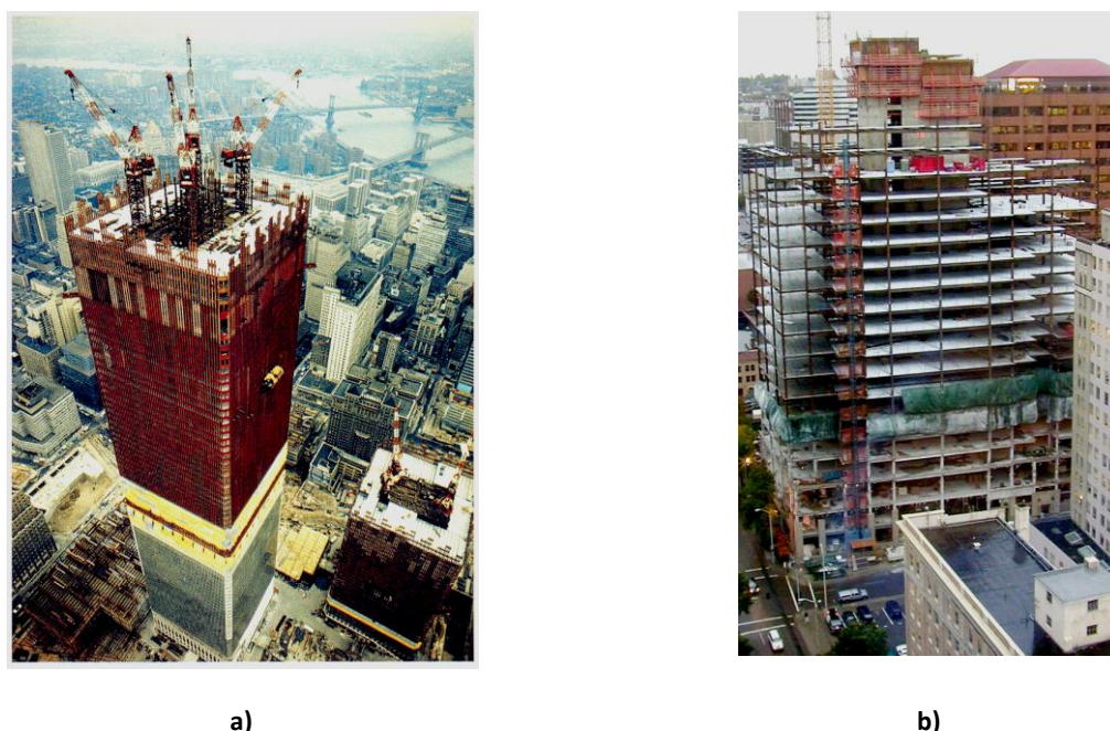
Figure 2.51 Construction of tall buildings: a) World Trade Center, New York, under construction 1971 showing exterior “tube” columns 43 , and b) high-rise under construction in Seattle, showing reinforced concrete shear wall around elevator core (Photo: C. Scawthorn)
