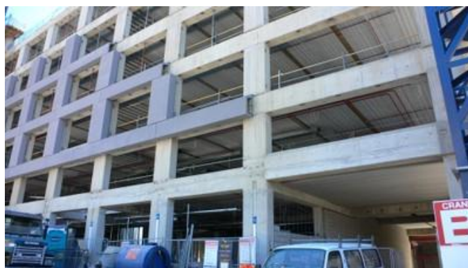
Figure 4.13 Reinforced concrete moment frame building, New Zealand (Photo: A. Charleson)
