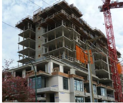
Figure 4.11 A reinforced concrete building with flat plate system in one direction and the wall system in other direction (Photo: S. Brzev)
