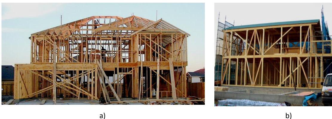
Figure 2.54 Modern wood frame construction: a) North American platform framing 46 , and b) Japanese house under construction, showing full story diagonal bracing (note, some bracing is only temporary) (Photo: C. Scawthorn)
