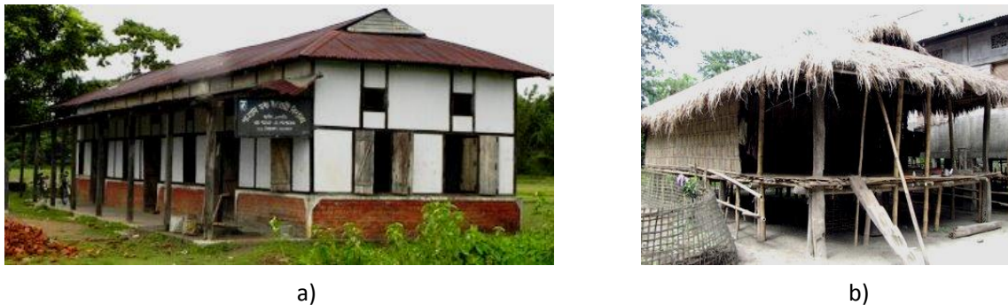
Figure 2.34 Lightweight vernacular buildings: a) Assam type building, India, and b) bamboo frame construction, India (Photos: People in Centre)
