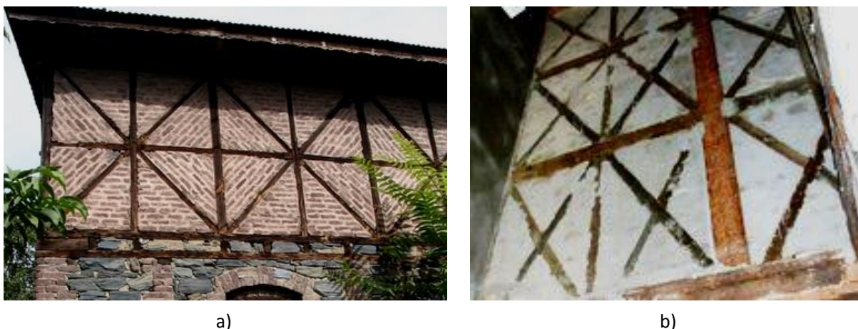
Figure 2.32 Composite timber and brick masonry construction: a) Dhajji Dewari , Kashmir, India, and b) a Pombalino building, Lisbon, Portugal (Photos: a) D. Rai, and b) S. Brzev)
