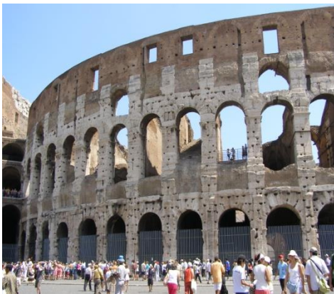
Figure 2.41 Arch structures: a) circular arches in Colosseum, Rome, and b) Arabic arches, Bara Gumbad Mosque, New Delhi, India (Photos: S. Brzev)
