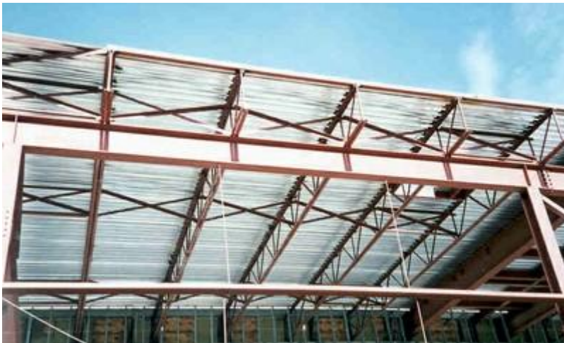
Steel trusses (open web steel joists) supporting corrugated steel roofing, Canada (S. Brzev)
