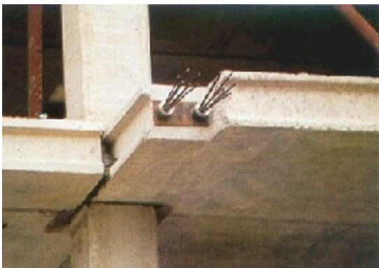
Precast prestressed concrete building under construction, showing precast slabs and columns, Serbia (R. Dimitrijevic)
