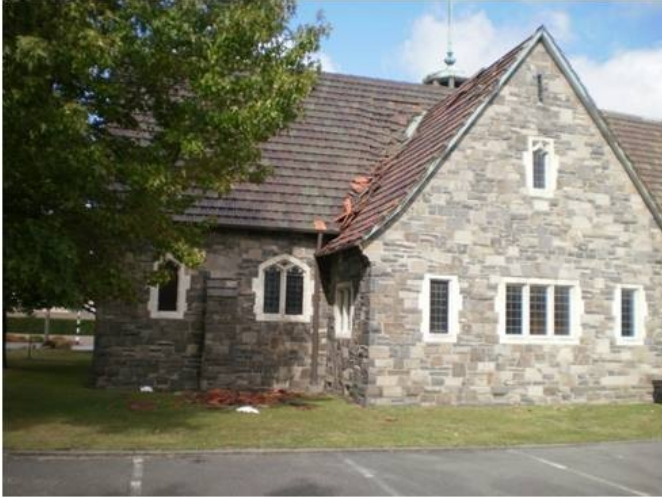
Stone masonry building - walls are likely to be a mix of basalt and trachyte stones with variation in block size and colour (J. Bothara)
