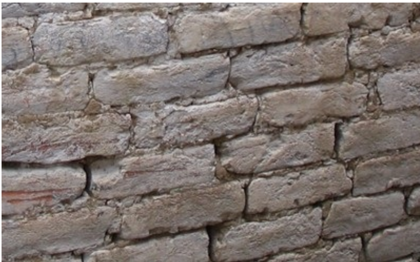
Mud mortar and fired clay bricks, India (D. Rai)
