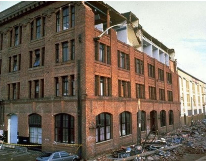
Out-of-plane collapse of masonry walls at the top floor level in a building due to inadequate roof-wall connection, 1989 Loma Prieta, California earthquake (EERI)
