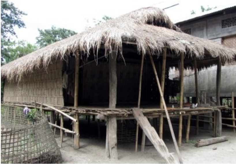
Bamboo frame construction on stilts found in flood- and earthquake-prone areas such as Assam, India (People in Centre)
