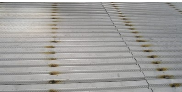
Steel decking joined by welds at regular spacing, Canada (S. Brzev)
