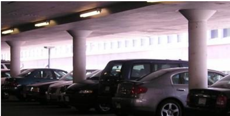
Reinforced concrete flat slab system (note column capitals), Vancouver, Canada (S. Brzev)
