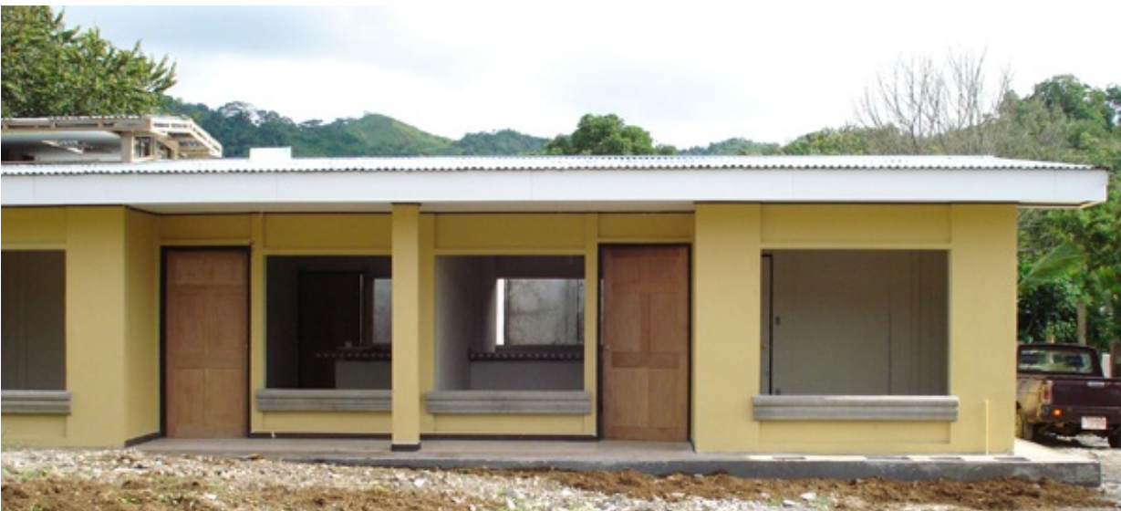
Large panel precast concrete construction, Kyrgyzstan (K. Kanbolotov)
