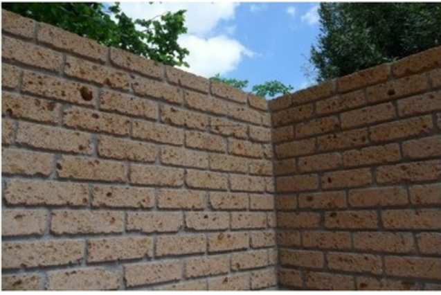
Tuff stone used in modern wall construction, Italy (A. Benedetti)
