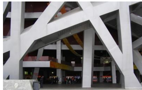
Birds Nest Stadium in Beijing, China has a 3-D braced frame structural system (S. Brzev)
