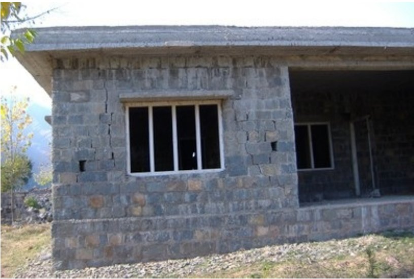
Reinforced concrete roof slab supported by walls, Pakistan (J. Bothara)
