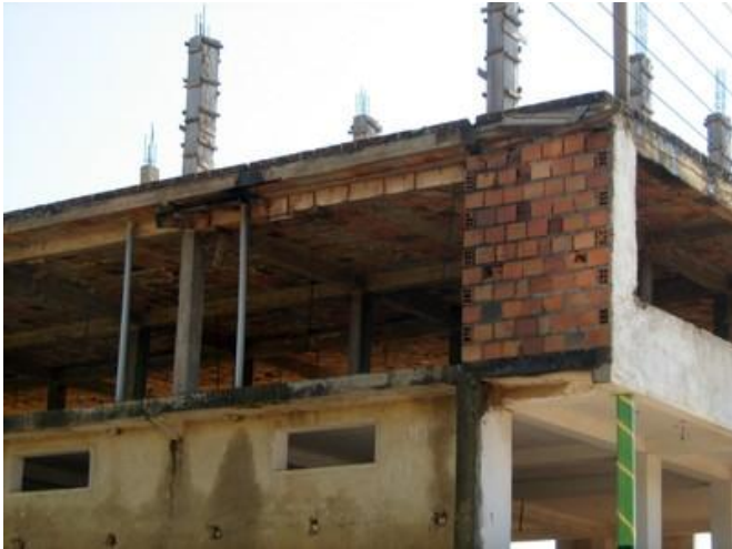
Reinforced concrete frame building with hollow clay block infills, Uganda (E. Lemkuhl)
