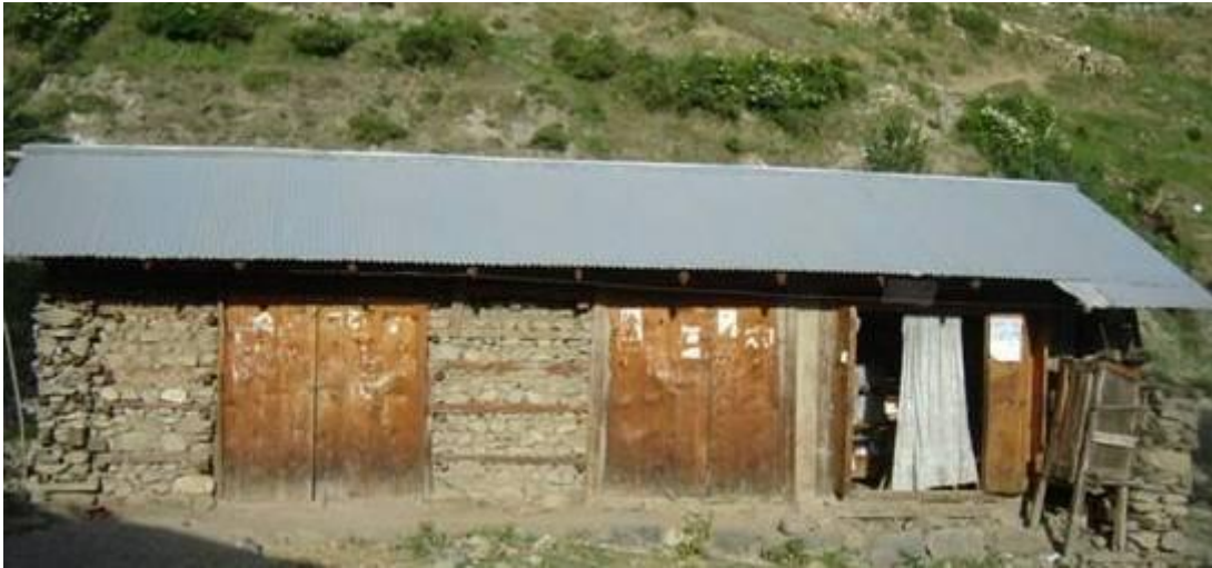
Rubble stone masonry with timber bands, NWFP, Pakistan (J. Bothara)
