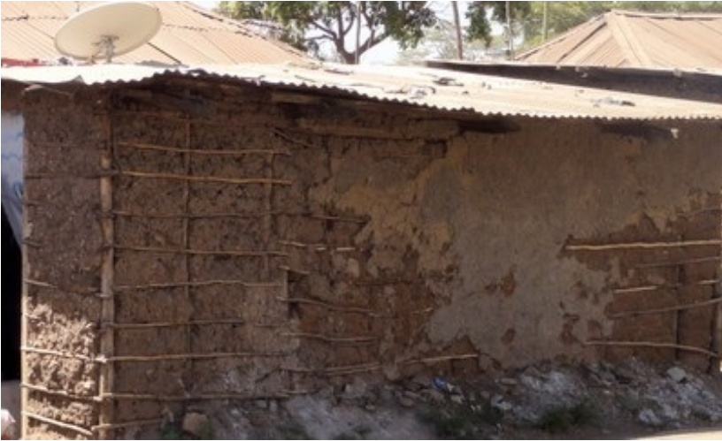
Mud wall with bamboo reinforcement, Kenya (K. Jaiswal)
