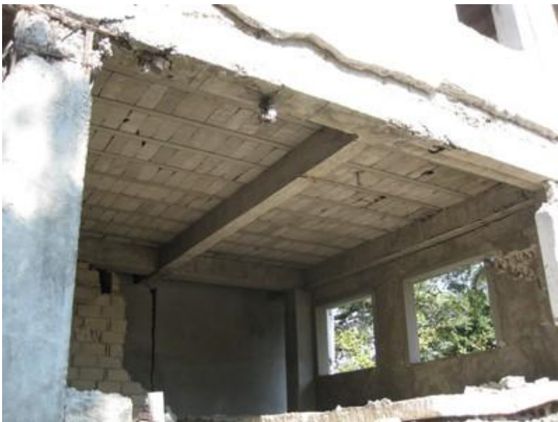
Floor system consisting of concrete masonry units and cast-in-situ reinforced concrete joists, Haiti (A. Lang)
