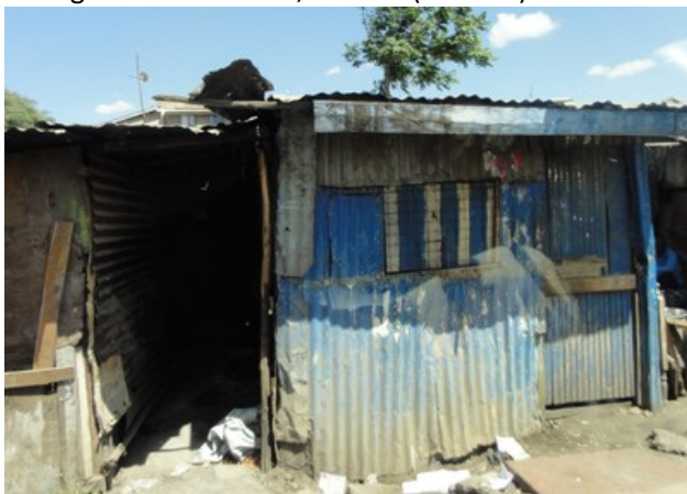
Exterior wall made of corrugated metal sheets, Kenya (K. Jaiswal)
