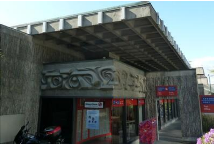
This reinforced concrete building has a waffle slab system, Vancouver, Canada (S. Brzev)
