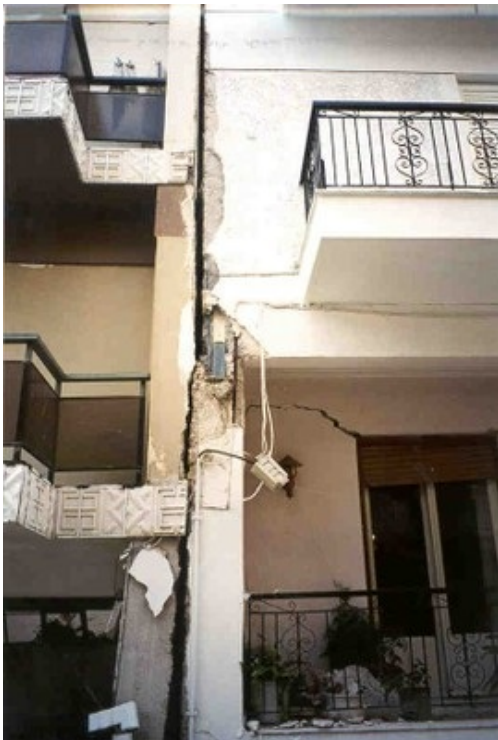
Damage due to pounding in reinforced concrete buildings with floors at different elevations in the 1999 Athens earthquake (A. Pomonis)
