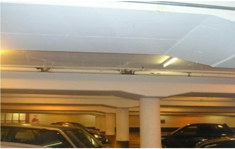
Reinforced concrete slab on beams in a parking garage, Canada (S. Brzev)
