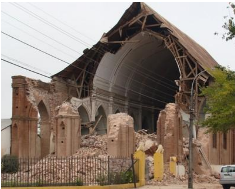
A church with a vaulted wooden roof in Curico, Chile damaged in the 2010 Maule, Chile earthquake (M.O. Moroni)
