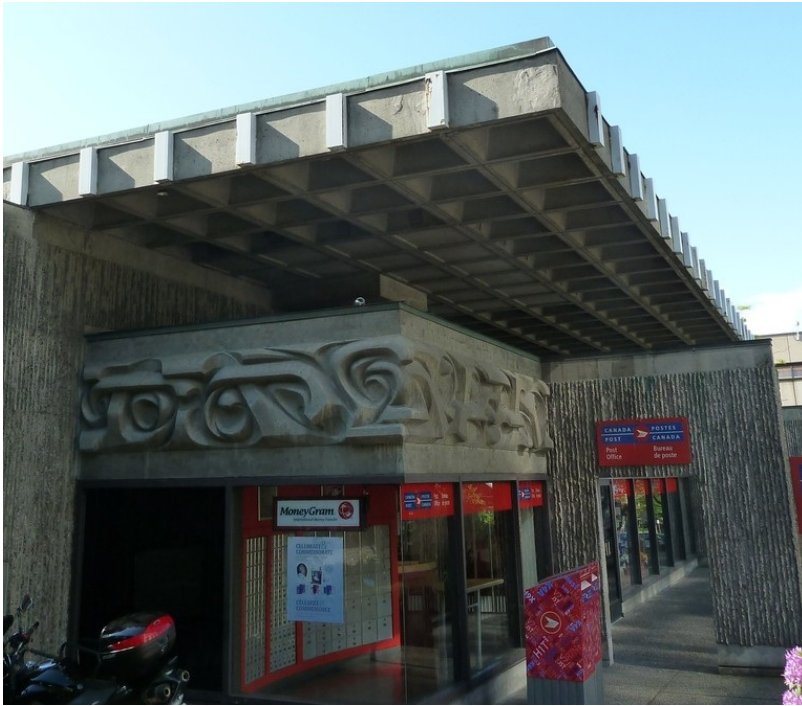
Waffle slab concrete construction, post office building, Canada (S. Brzez)
