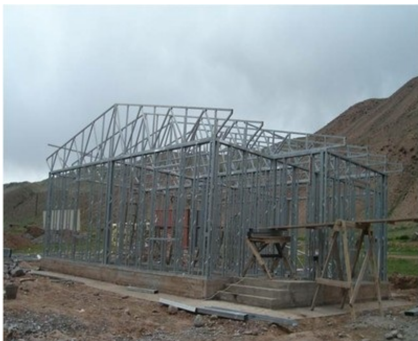
Cold formed steel construction, Kyrgyzstan (K. Kanbolotov)
