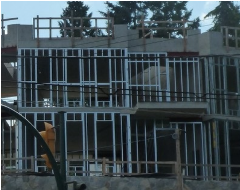
Cold-formed steel framing, Canada (S.Brzev)
