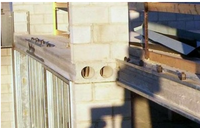
Precast concrete hollow floor slab supported by concrete block masonry walls, Canada (J. Adams)
