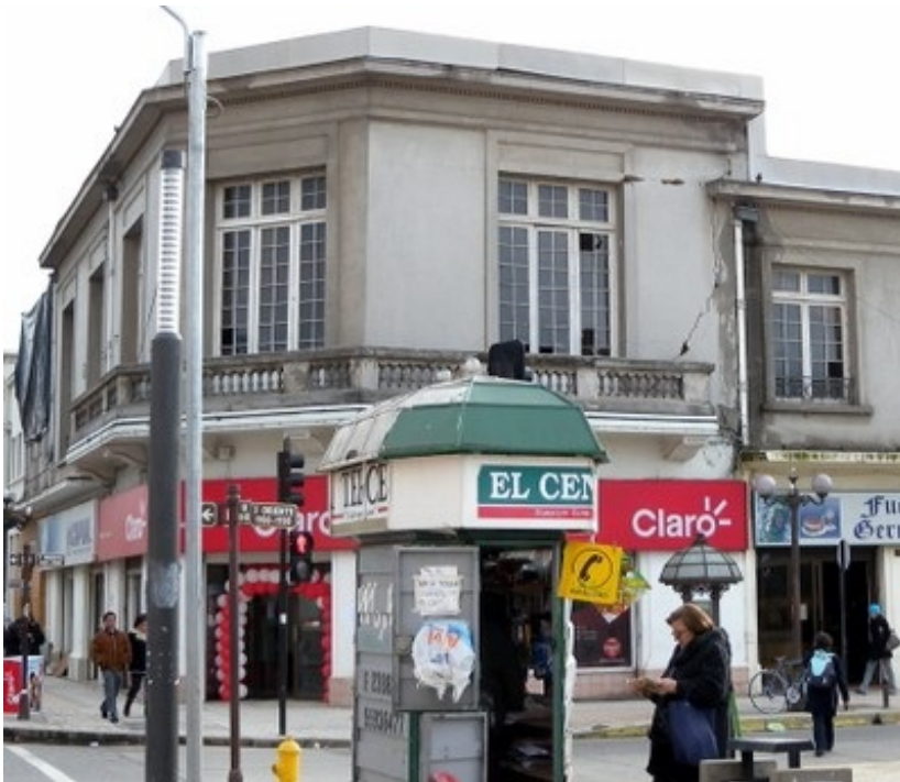
Pounding damage due to the 2010 Chile earthquake (S. Brzev)
