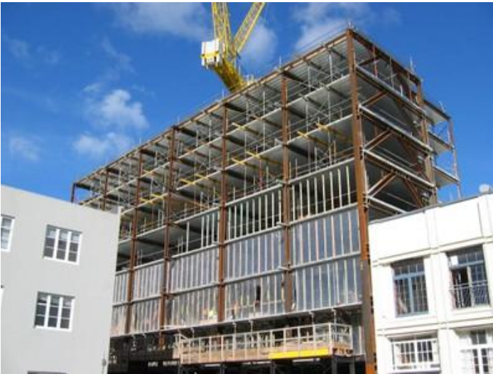
Eccentrically braced steel frame under construction, New Zealand (A. Charleson)
