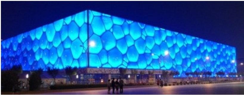
National Swimming Center in Beijing, China (also known as The Cube) is a space (3-D) frame assembled from 22,000 steel tubes welded to 12,000 nodes; this is a unique structure (D. Willms)
