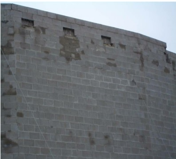
Out-of-plane collapse of masonry walls in a building damaged in the 1994 Northridge, California earthquake; note floor-wall anchors (EERI)
