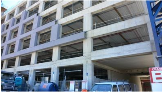
Moment frame, concrete, New Zealand (A. Charleson)
