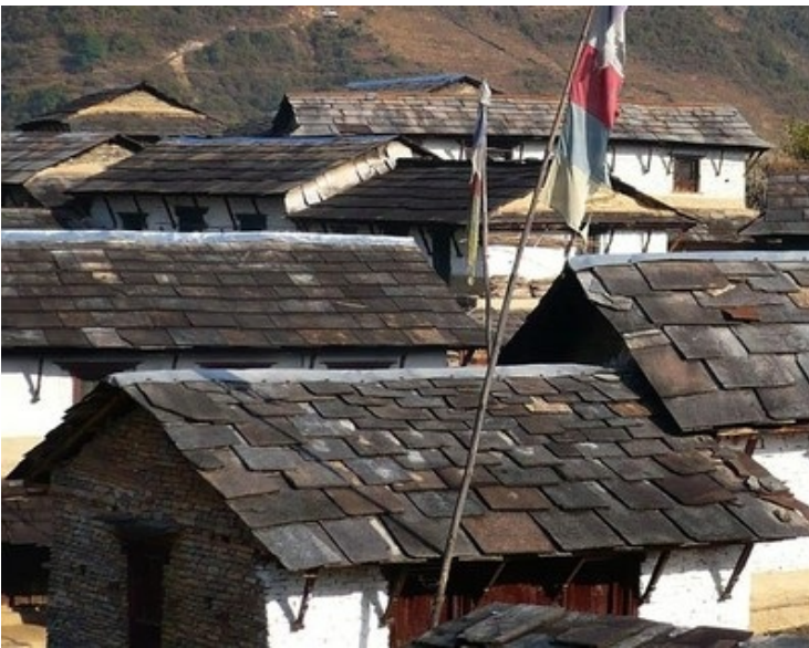
Wooden roof structure with stone slate tiles, Nepal (M. Schildkamp)
