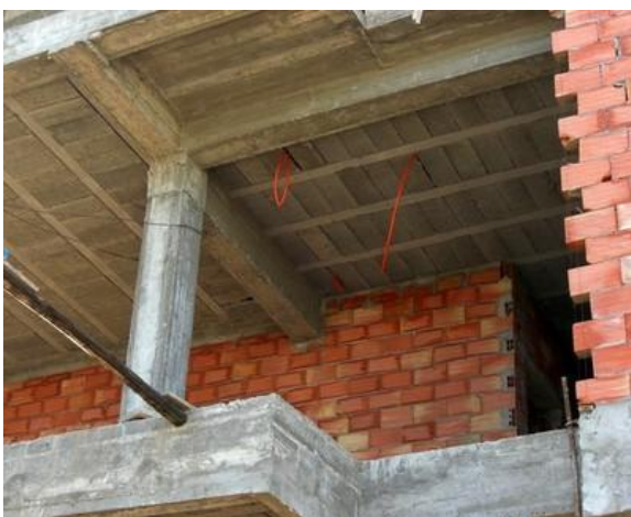
Detail of a reinforced concrete frame with hollow clay tile infill, Rabbat, Morocco (C. Scawthorn)
