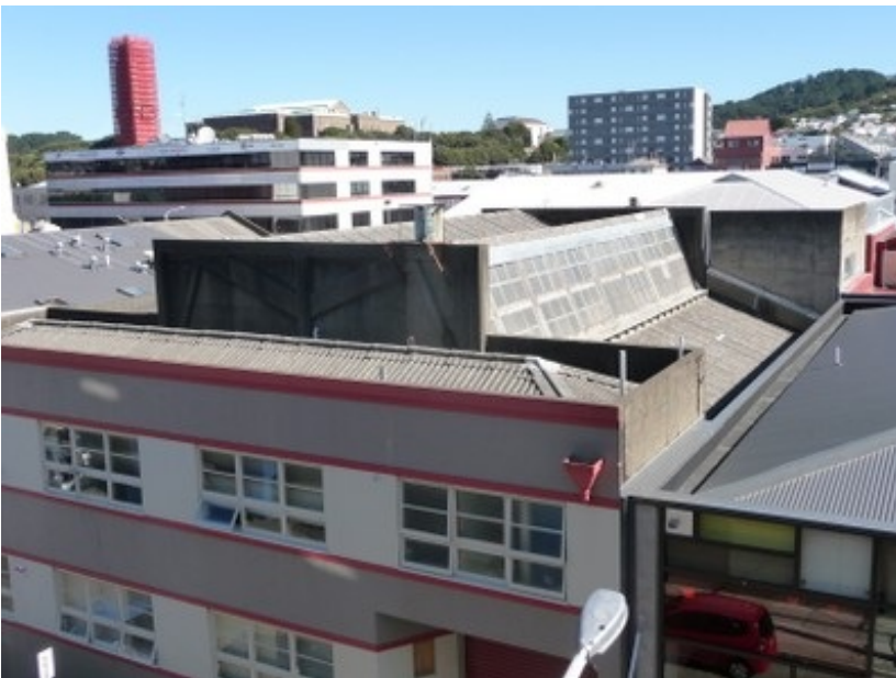
An irregular roof, an arrangement of multiple roof shapes and pitches on a single building, New Zealand (A. Charleson)
