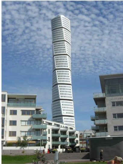
HSB Turning Torso in Malmö, Sweden has aluminum exterior walls (C. Scawthorn)
