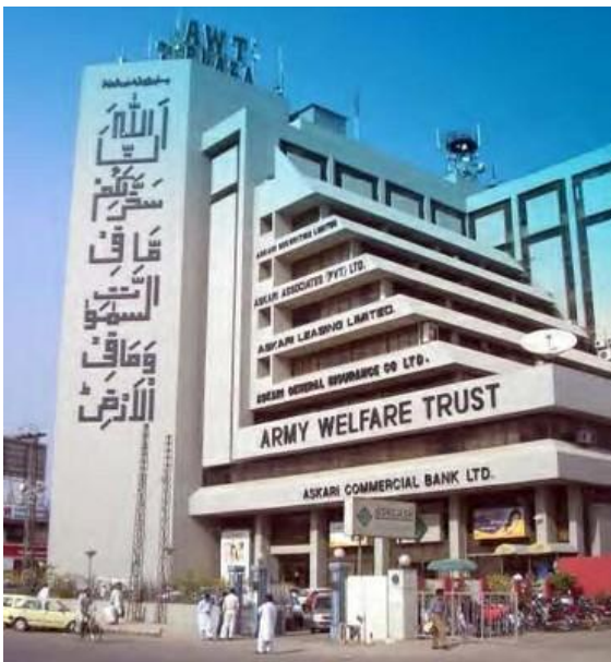
This building in Rawalpindi, Pakistan is characterized by a change in vertical structure and it suffered damage in the 2005 Kashmir earthquake (C. Scawthorn)
