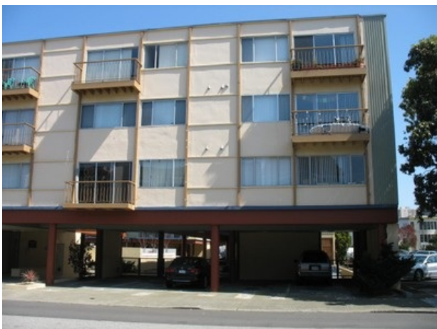
A hybrid system consisting of cast-in-place reinforced concrete frame construction at the ground floor level and wood frame construction above can be found in California (USA) and British Columbia (Canada) (D. Bonowitz)
