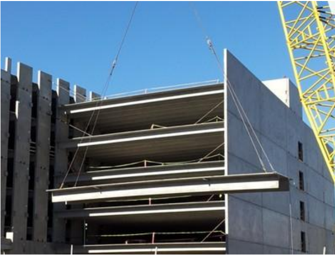
A double-tee beam lifted by the crane at the construction site, Denver, USA (K. Porter)
