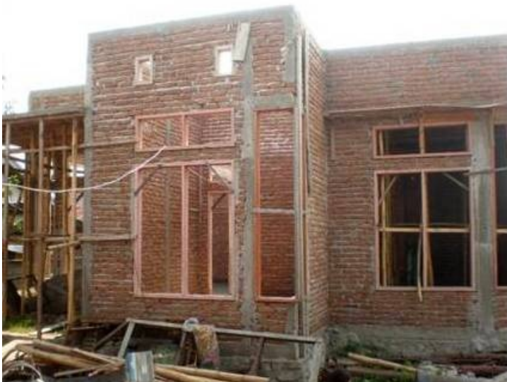
Confined masonry construction, Indonesia (J. Bothara)
