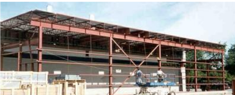
Concentrically braced steel frame under construction, Canada (S. Brzev)
