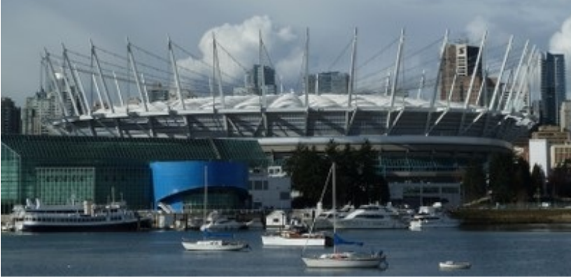
BC Place Stadium in Vancouver, Canada has a tensile membrane roof; the roof is covered by a semi-transparent plastic material (ETFE) (S. Brzev)
