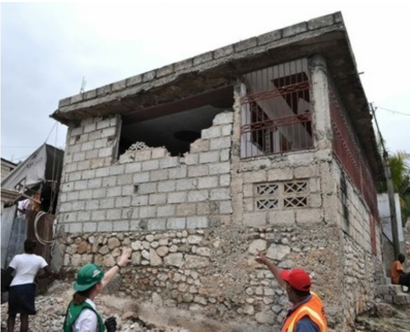
Damage of a poorly constructed confined masonry building in the 2010 Haiti earthquake; this is considered a non-ductile performance (A. Lang, EERI)
