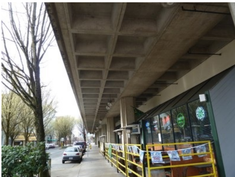
Reinforced concrete waffle slab system with beams, USA (S. Brzez)
