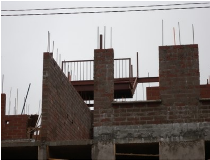
Reinforced clay block masonry, Chile (S. Brzev)
