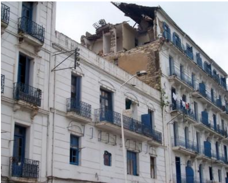
Stone masonry building in Algiers suffered damage in the 2003 Boumerdes, Algeria earthquake (M. Farsi)
