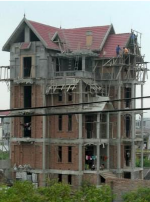
Reinforced concrete frame with masonry infills under construction, Vietnam (C. Scawthorn)
