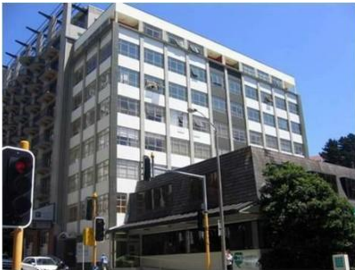
A 1970s reinforced concrete frame, Wellington, New Zealand (J. Bothara)
