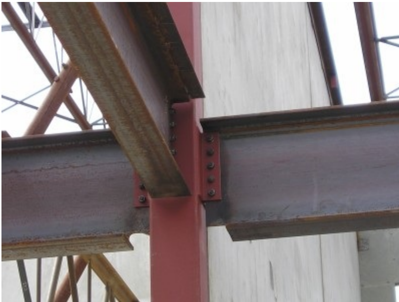
Bolted connection of three steel members joined at a column, Canada *S. Brzev)
