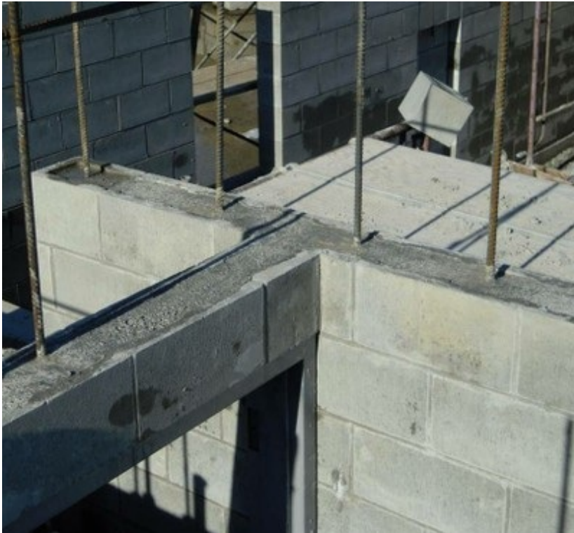
Concrete block masonry construction with steel reinforcement, Canada (B. McEwen)
