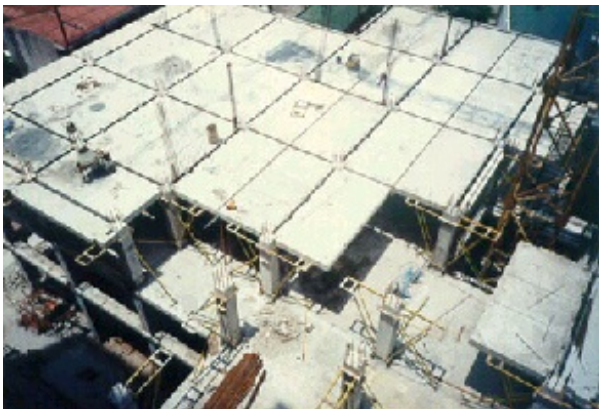
Precast prestressed concrete building under construction, showing precast slabs and columns, Serbia (R. Dimitrijevic)
