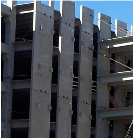
Wall corbels ready to support double-tees, Denver, USA (K. Porter)
