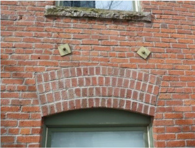
A retrofitted unreinforced brick masonry building with floor-wall anchors visible at the exterior, Vancouver, Canada (S. Brzev)
