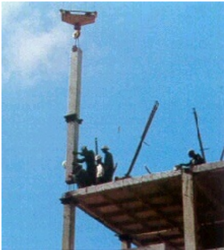
Erection of precast concrete columns, Serbia (R. Dimitrijevic)
