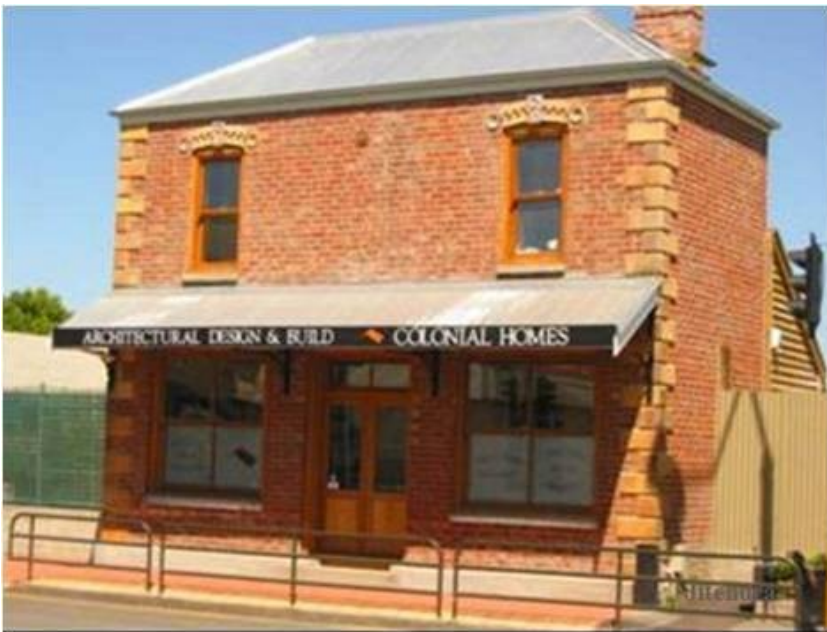
Clay brick masonry in cement:sand mortar, Christchurch, New Zealand (J. Bothara)
