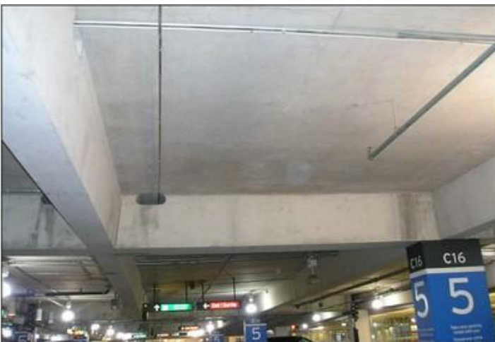
Reinforced concrete buildings with a moment frame system have beams as a part of the floor system (Canada, S. Brzev)
