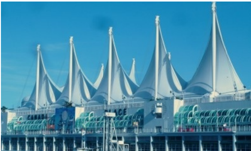
Canada Place in Vancouver, Canada is an example of tensile fabric roof structure (S. Brzev)
