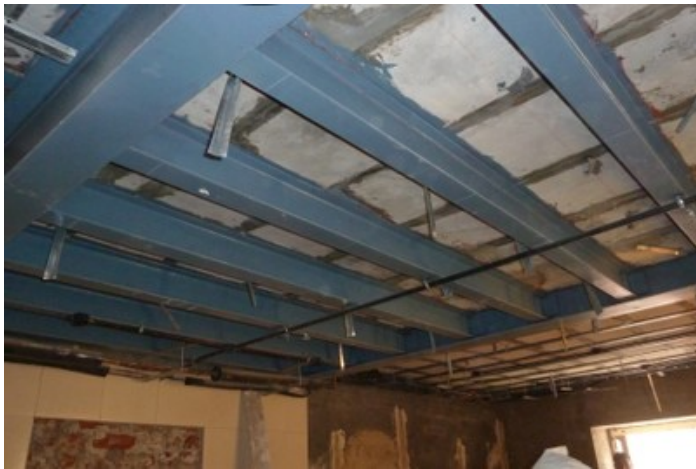
Metal beams supporting precast concrete slabs, India (S. Brzev)
