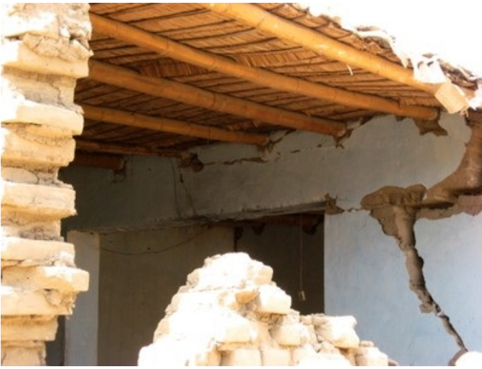
Typical flat roof found in adobe buildings in Peru made of wooden (or bamboo) beams overlaid with straw, mud, and in some cases tiles or metal sheets (N. Tarque)
