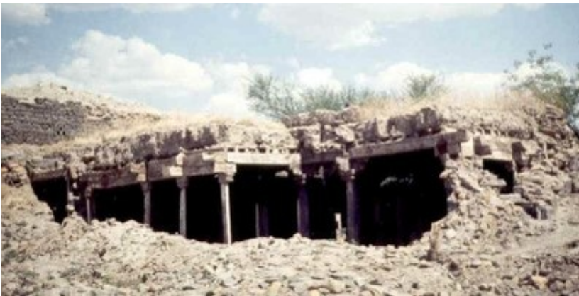
Wooden roof with a heavy mud overlay caused many fatalities in the 1993 Maharashtra, India earthquake (S. Brzev)
