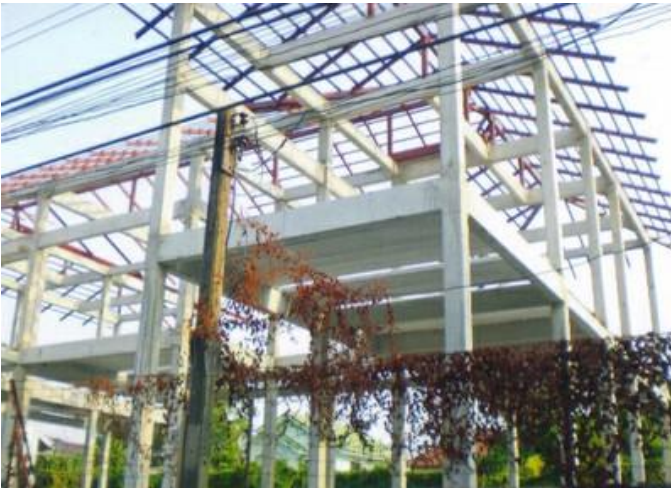
Reinforced concrete frame under construction, Thailand (C. Lilavivat)
