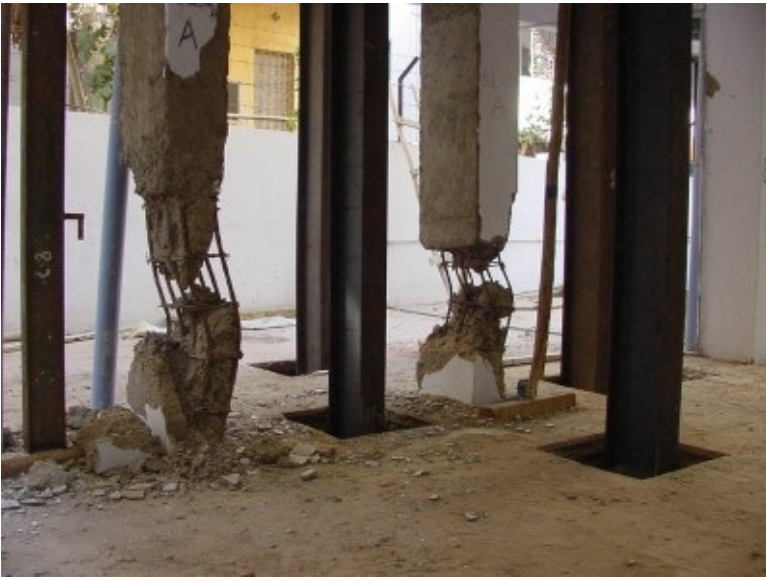
Ties in reinforced concrete columns: a) 135 degree hooks (ductile detailing), and b) 90 degree hooks (non-ductile detailing) (Brzev, S. and Pao, J. Reinforced Concrete Design: A Practical Approach , Pearson Learning Solutions, 2012)
