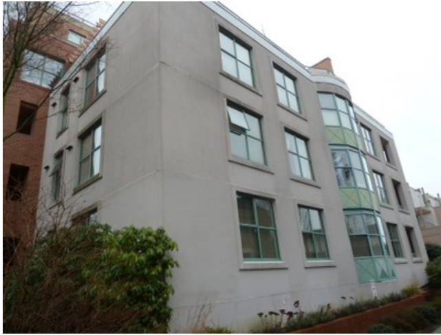
Stucco cladding over wood stud walls, Canada (S. Brzev)
