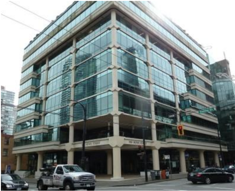
Flat slab structure, Canada - note column capitals (S. Brzev)
