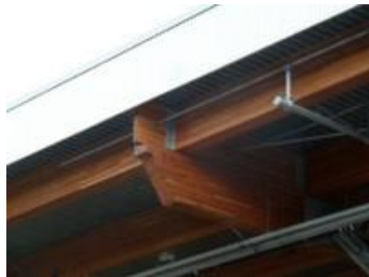
A roof structure consisting of steel decking supported by wooden glulam beams, Vancouver, Canada (S. Brzev)
