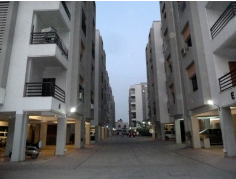
Soft storey in reinforced concrete buildings, India (S. Brzev)
