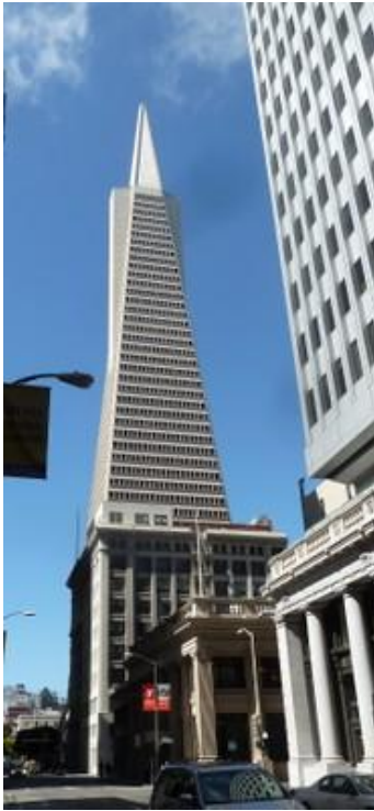
Transamerica Pyramid, the tallest skyscraper in San Francisco, California is characterized by a change in vertical structure (S. Brzev)
