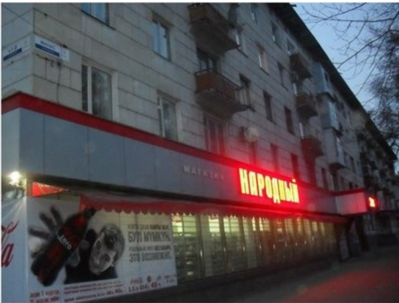
Buildings with a cast in-situ reinforced concrete frame at the ground floor level and brick masonry or concrete walls above can be found in Kyrgyzstan (K. Kanbolotov)
