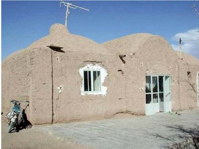
Earthen roof covering, Iran (F. Naeim, World Housing Encyclopedia Report 104)
