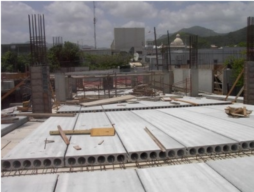
Precast concrete hollow core slabs (tropicalconcrete.com)
