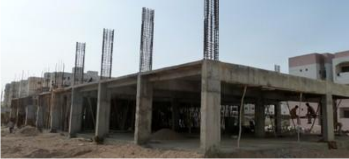
Reinforced concrete frame building under construction, India (S. Brzev)
