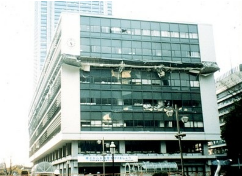
Collapse of the 6th storey of the 8-storey Kobe City Hall Annex building in the 1995 Kobe, Japan earthquake. The collapse was likely due to a hybrid lateral load-resisting system consisting of steel reinforced concrete (SRC) at lower floors and RC frame at upper floors (C. Scawthorn).
