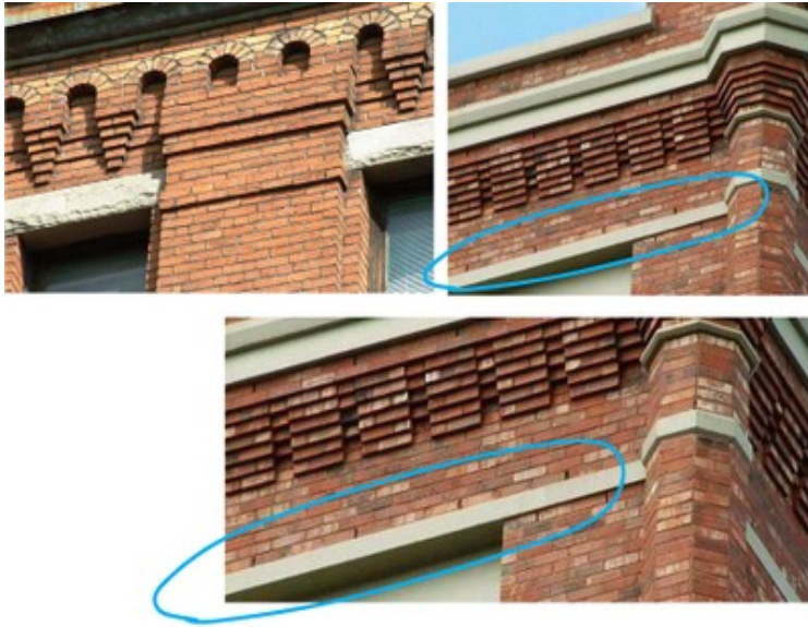
The exterior walls shown on the top photos look like loadbearing brick masonry construction. The photo on the left shows an older loadbearing brick masonry wall (built between 1900 and 1950), while the photo on the right shows a wall in a modern building (built between 1990 and 2010) which has similar masonry detailing like older buildings. However, the exterior brick masonry wall is a veneer and the loadbearing wall is likely a wood frame. The wall has weep holes characteristic of veneer construction (see detail on the bottom photo). The photos were taken in Vancouver, Canada (B. McEwen)
