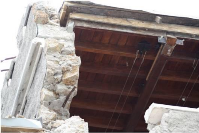
Timber beams and joists supporting light roofing, New Zealand (W. Clark)
