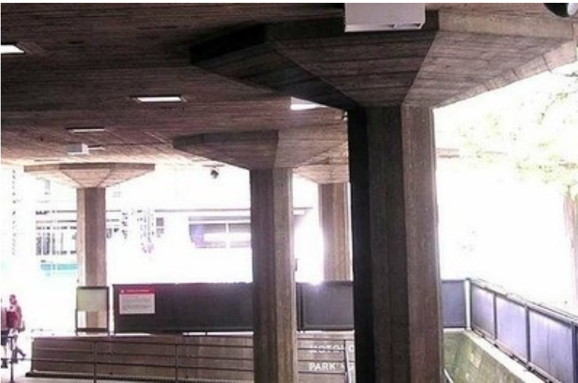
Reinforced concrete flat slab system with capitals, UK (S. Brzev)
