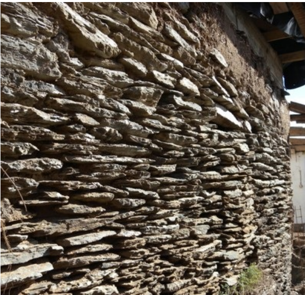
Slate stone used for wall construction in coastal areas of Chile (S. Brzev)
