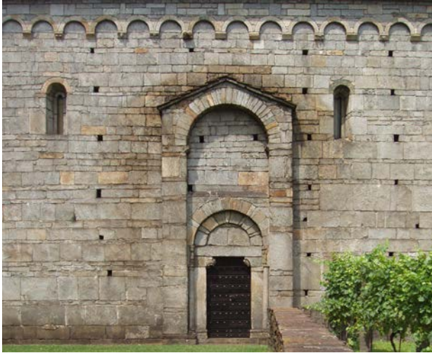
Gneiss stone walls, a 12th century church, Ticino, Southern Switzerland (T. Schacher)
