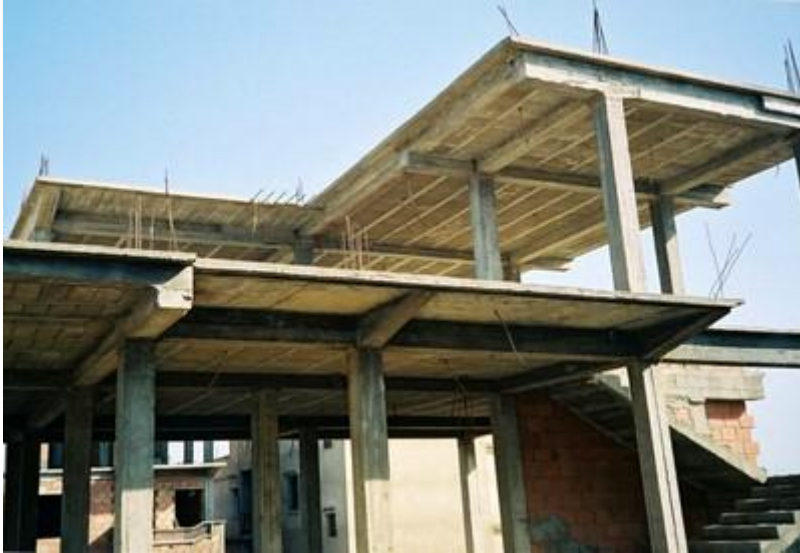
Roof/floor system consisting of cast-in-place reinforced concrete joists and precast concrete masonry units, Algeria (S. Brzev)
