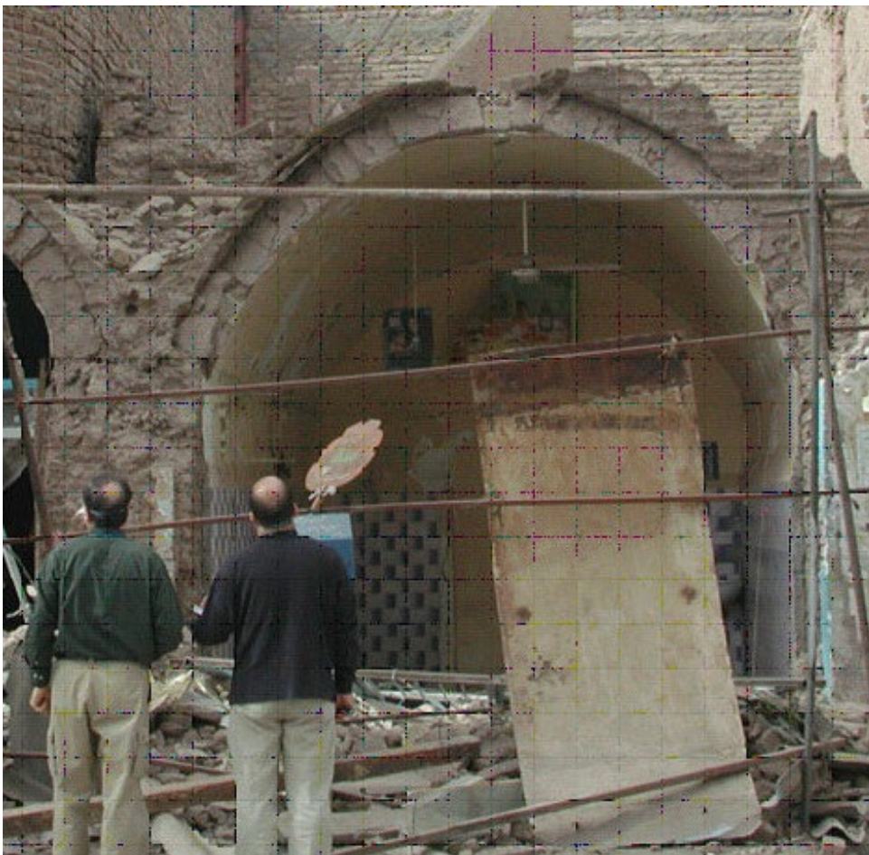
Collapse of earthen buildings with domed roofs in the 2003 Bam, Iran earthquake (F. Naeim)
