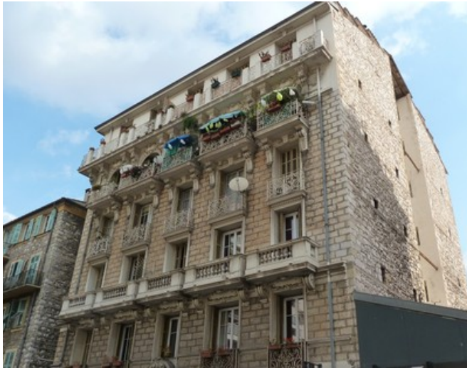
Stone masonry walls: dressed stone at the front facade and uncoursed stone masonry in the perpendicular direction, France (S. Brzev)
