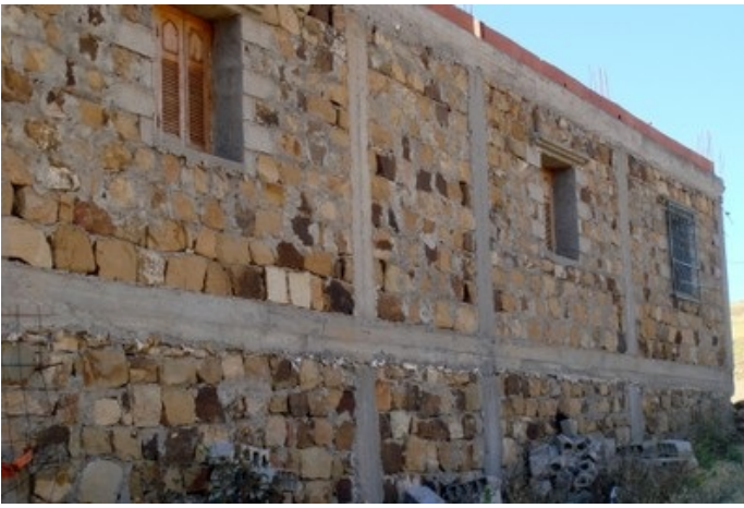
Confined stone masonry construction, Algeria (M. Farsi)
