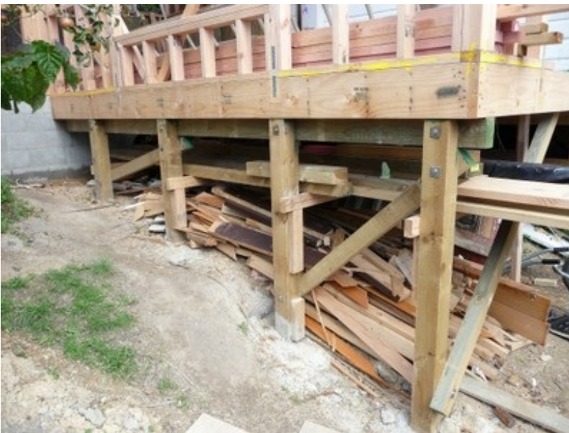
Examples of braced timber pile foundations, New Zealand (Charleson).
