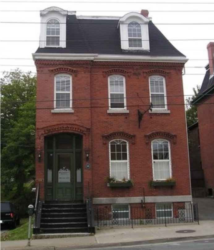
A typical unreinforced masonry building from the beginning of 20th century, Halifax, Canada (S. Brzev)
