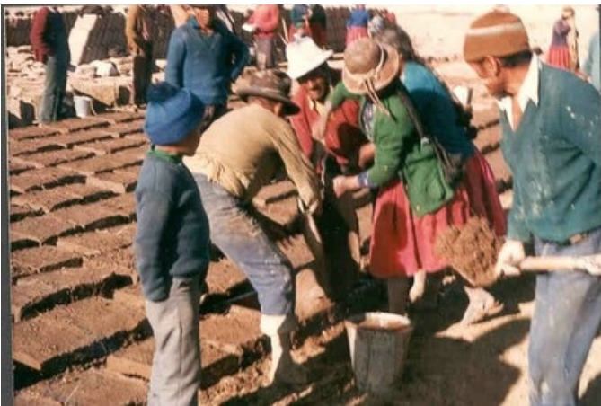
Manufacturing of adobe blocks, Peru (left - M. Blondet) and different sizes of adobe blocks (right- S. Brzev)
