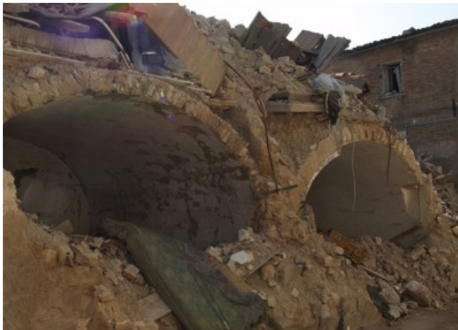
Damage to masonry buildings with vaulted masonry roofs in L'Aquila earthquake, Italy (T. Schacher)
