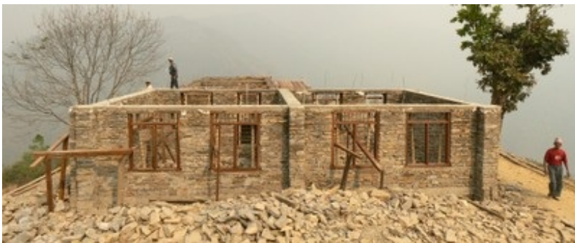
Stone masonry building with a reinforced concrete band at lintel level, Nepal (M. Schildkamp)
