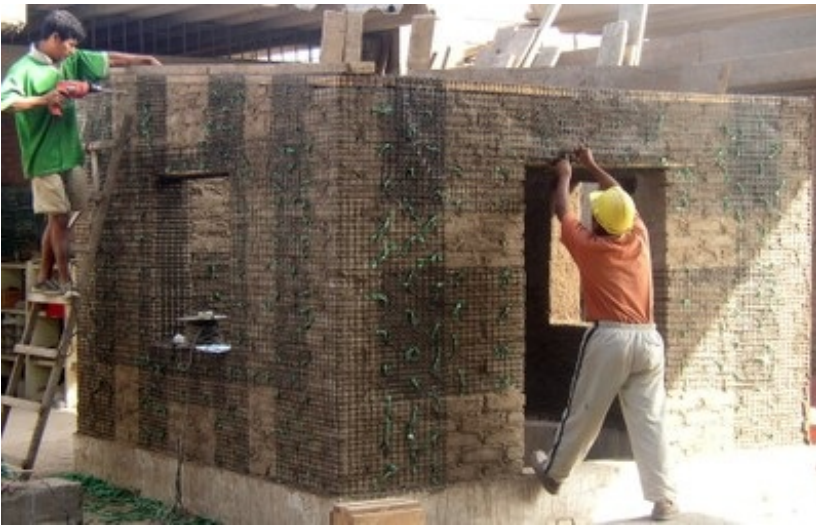
Adobe walls reinforced with a polymer mesh (geogrid) attached to the walls by plastic or nylon strings, Peru (N. Tarque)
