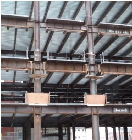
Steel beams supporting composite steel and concrete deck floor, USA (S. Brzev)
