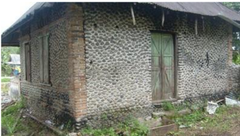
Rubble stone masonry constructed using round river stones in lime or cement:lime mortar, usually 250 mm thick, West Sumatra, Indonesia (J. Bothara)
