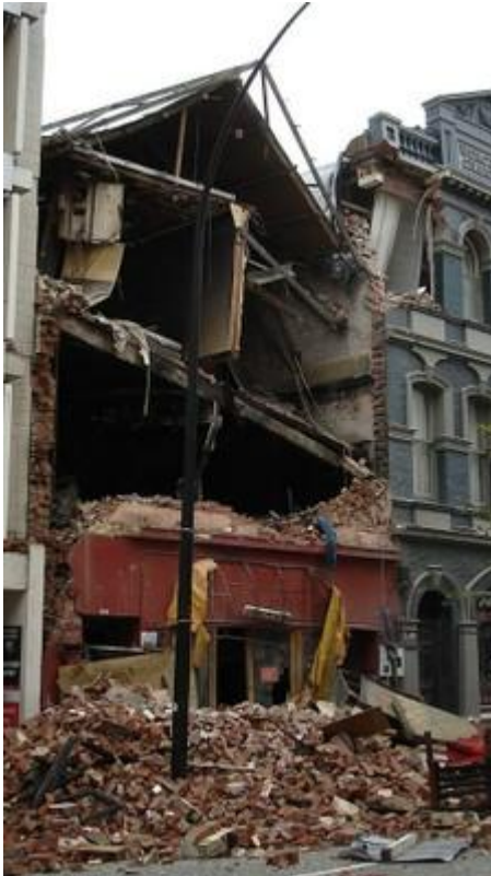
Out-of-plane wall collapse was reported in some unreinforced masonry buildings due to the 2011 Christchurch, New Zealand earthquake; the building shown on the photo had inadequate floor-wall connections (K. Elwood)
