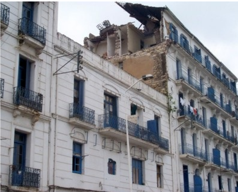
Tuff stone masonry in Algiers, Algeria was affected by the 2003 Boumerdes earthquake (M. Farsi)
