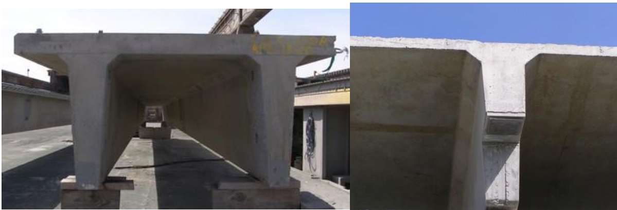
A typical double-tee element (left) and the end support (right) (S. Brzev)
