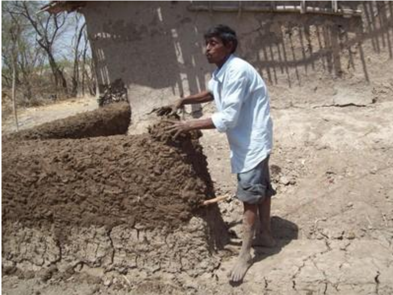
A cob wall under construction, India (People in Centre)
