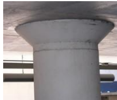
Reinforced concrete flat slab system (note column capitals), Vancouver, Canada (S. Brzev)
