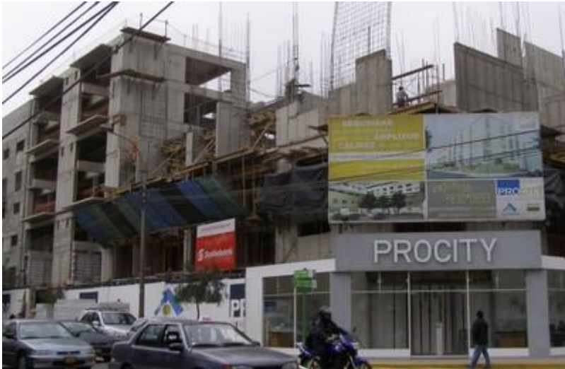
Reinforced concrete wall building under construction, Lima, Peru (S. Brzev)
