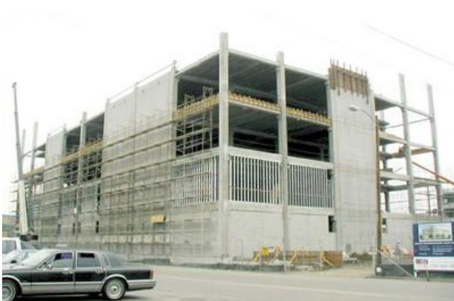
A cast-in-place reinforced concrete building with a Wall lateral load-resisting system, Oakland, California, USA (C. Scawthorn)
