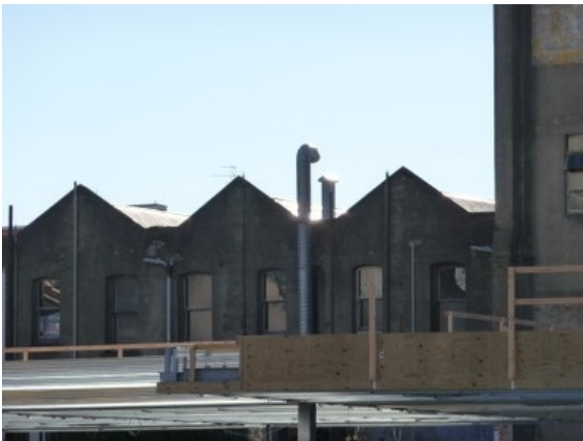
Complex regular roof, a repeating arrangement of multiple pitched gable roofs, New Zealand (A Charleson).
