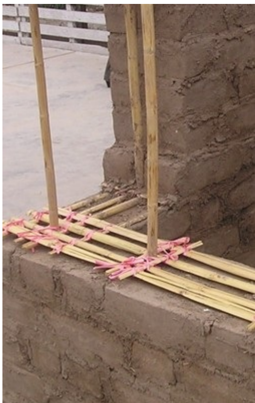
Adobe wall with cane reinforcement, Peru (S. Brzev)
