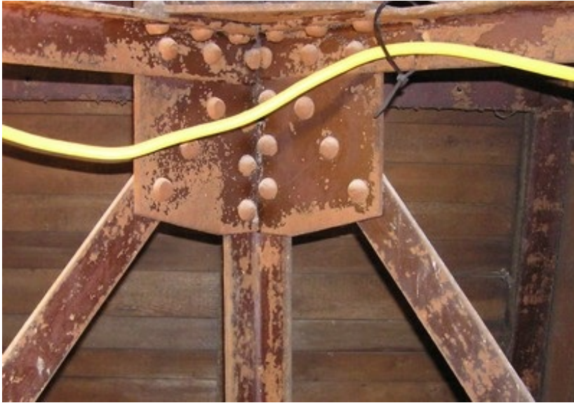
Riveted connection, Canada (Ojdrovic Engineering)
