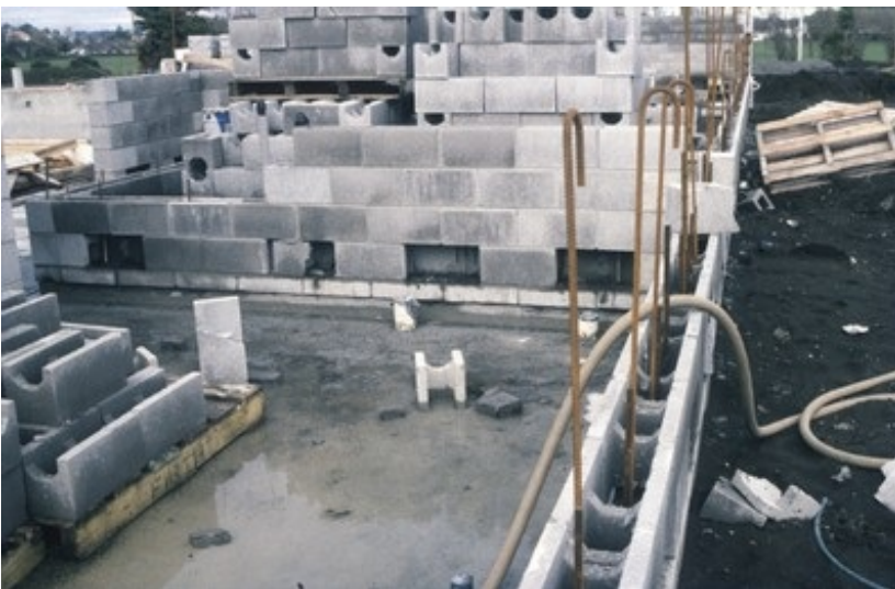
Reinforced concrete block masonry, New Zealand - note vertical reinforcing bars placed in hollow cores (A. Charleson)
