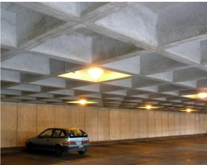
A reinforced concrete waffle slab, Eugene, USA (S. Brzev)
