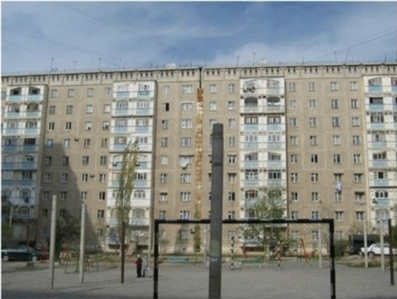
Large panel precast concrete construction, Kyrgyzstan (K. Kanbolotov)
