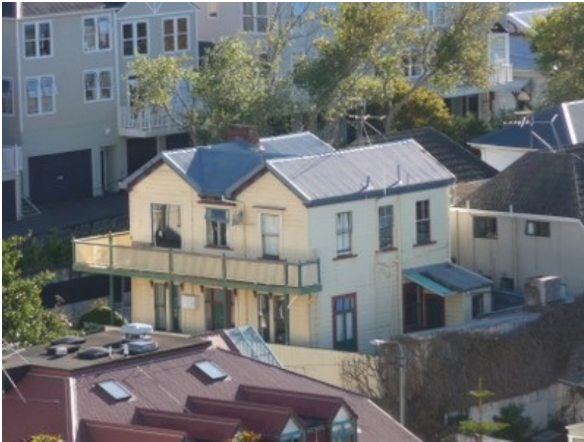
Complex regular roof, a symmetrical arrangement of multiple pitched gable roofs, New Zealand (A Charleson).
