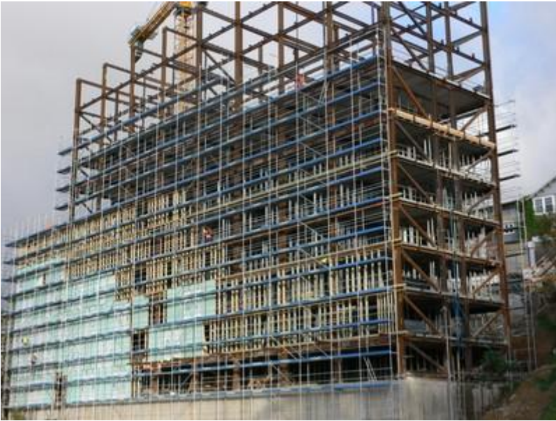
Steel building construction, hot-rolled steel members, Wellington, New Zealand (A. Charleson)
