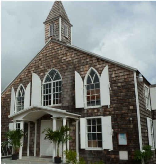
Wood shingles cladding, Saint Martin (Caribbean) (S. Brzev)
