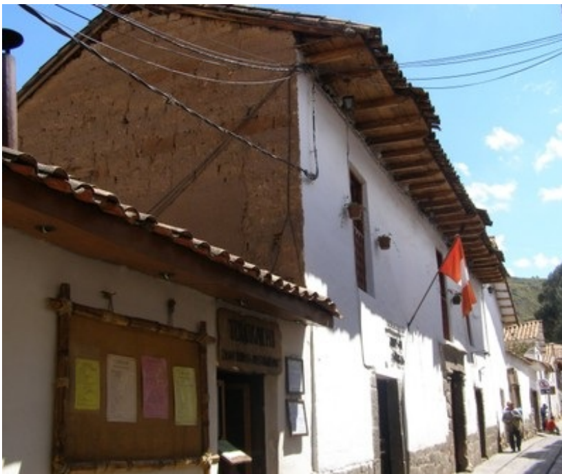
Tw-storey adobe building in Cuzco, Peru (S. Brzev)
