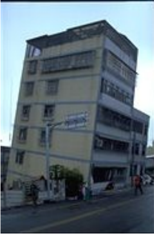
Building with an open first storey along street corner and walls along other exterior faces collapsed in the 1999 Chi Chi, Taiwan earthquake. The building tilted due to collapse of first storey columns, creating apparent torsional weakness (Courtesy of the NISEE, University of California, Berkeley, photo: J. Moehle)
