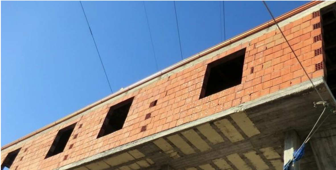
Fired clay tile masonry wall construction, Albania (C. Scawthorn)
