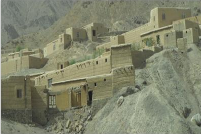
Rammed earth construction in Bamyan Province, Afghanistan (Aga Khan Development Network)
