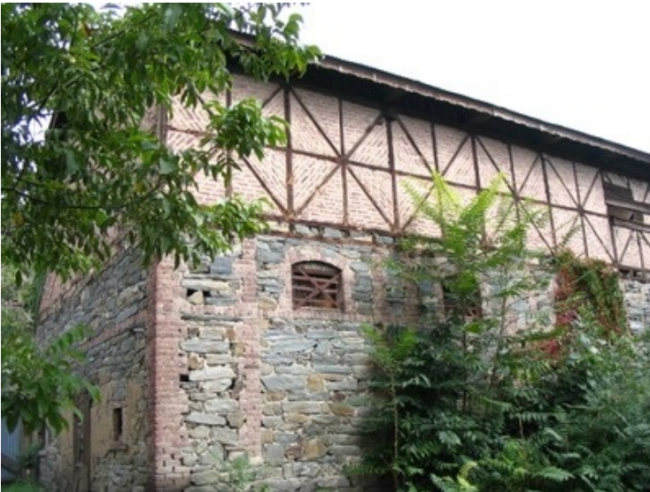
A building with the ground floor consisting of unreinforced stone and brick masonry construction, and the second storey with Dhajji Dewari construction, Kashmir, India (D. Rai)
