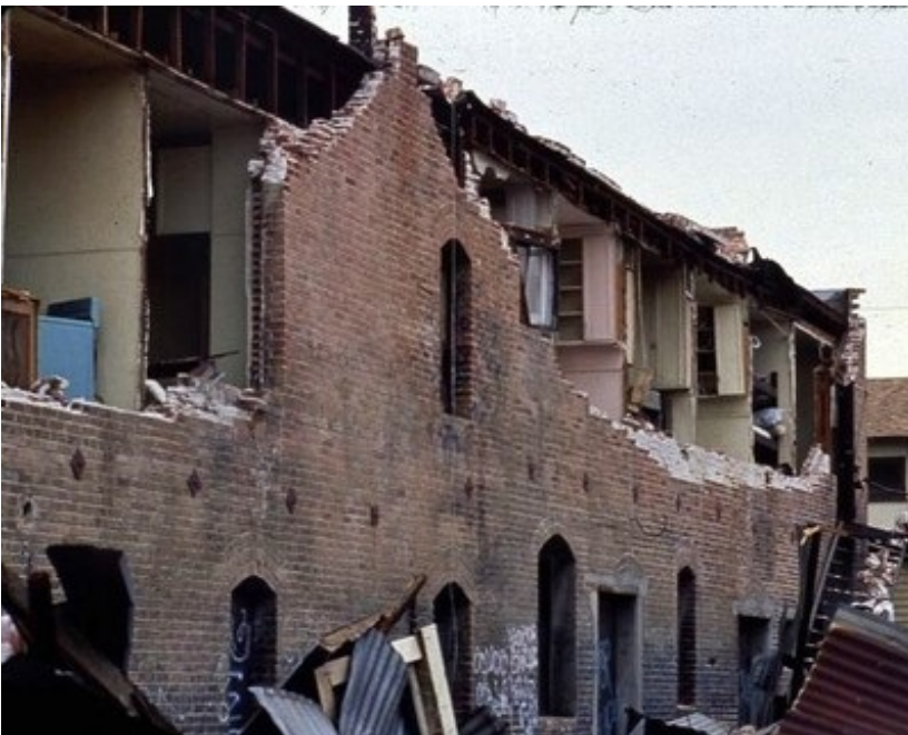
Out-of-plane collapse of masonry walls in a building damaged in the 1994 Northridge, California earthquake; note floor-wall anchors (EERI)
