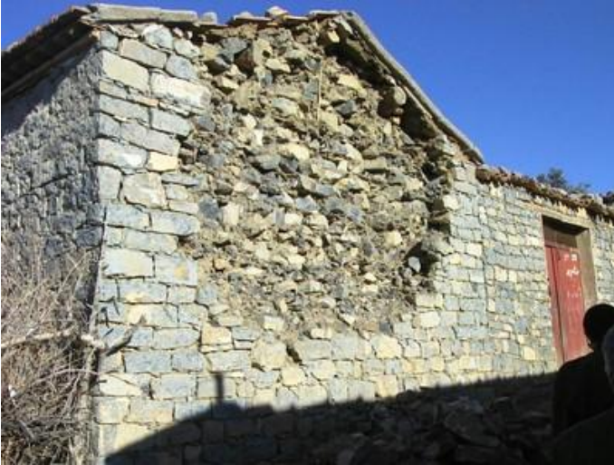
Limestone masonry wall in Beni-Ourtlane damaged in the 2000 earthquake (M. Farsi)
