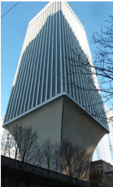
Change in vertical structure, Seattle, USA (S. Brzev)
