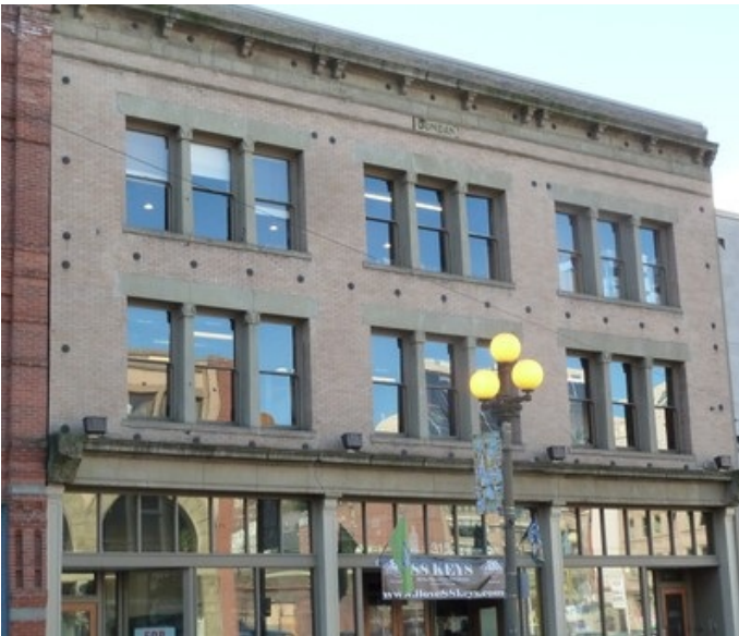
A retrofitted unreinforced brick masonry building showing exposed floor-wall and roof-wall anchors at the exterior, Seattle, USA (S. Brzev)
