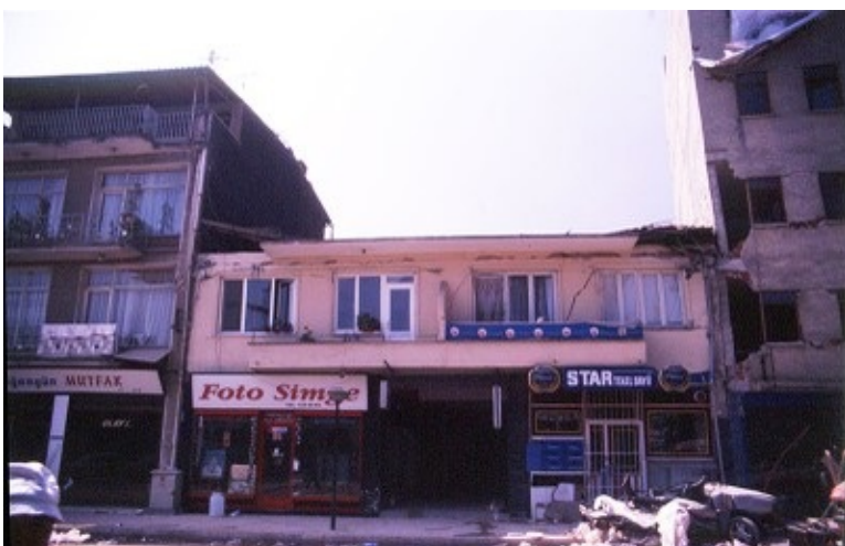
Damage due to pounding in reinforced concrete buildings with floors at different elevations in the 1999 Athens earthquake (A. Pomonis)
