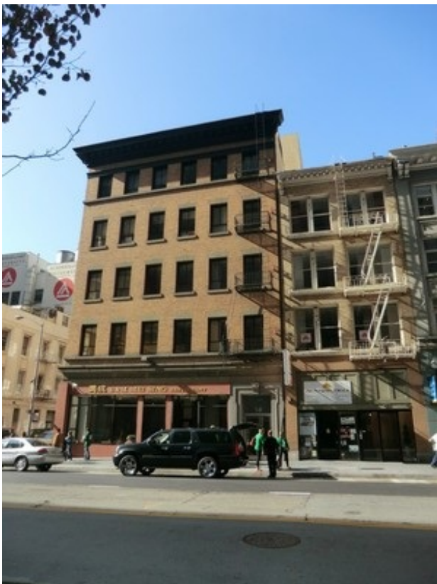
Adjacent buildings of different height without seismic gap, pounding potential, San Francisco, USA (C. Scawthorn)
