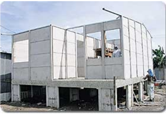
Precast concrete construction technology comprising horizontal wall panels and vertical posts and is used for one-storey housing, Costa Rica (A. Cuevas Ramirez)
