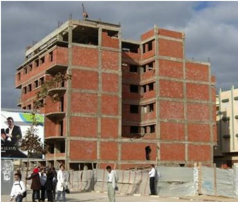
Reinforced concrete frame with masonry infills, Tangier, Morocco (C. Scawthorn)
