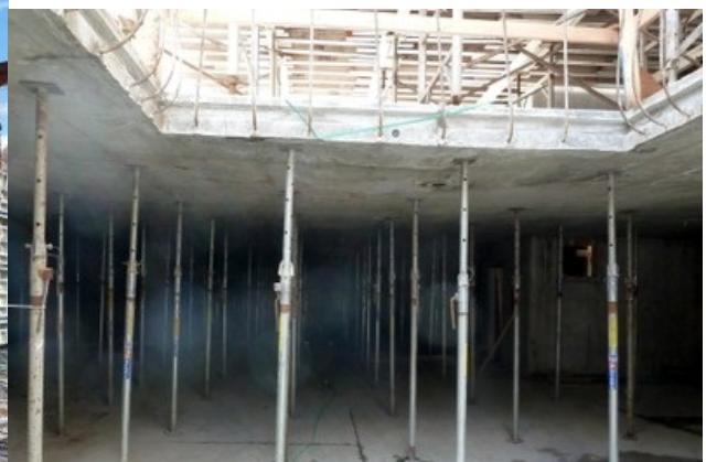
Cast-in-place concrete beam construction (note reinforcement and formwork), Canada (S. Brzev)
