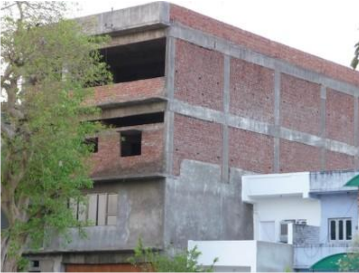
Reinforced concrete frame with brick masonry infill walls, India (A. Charleson)
