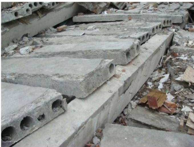
Concrete floors consisting of hollow core slabs with inadequate connections collapsed in the 2008 Wenchuan, China earthquake (J. Dai)
