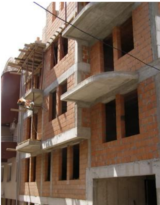
Hollow clay tile masonry construction, Belgrade, Serbia (S. Brzev)
