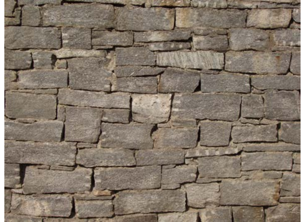
Gneiss stone walls, a 12th century church, Ticino, Southern Switzerland (T. Schacher)
