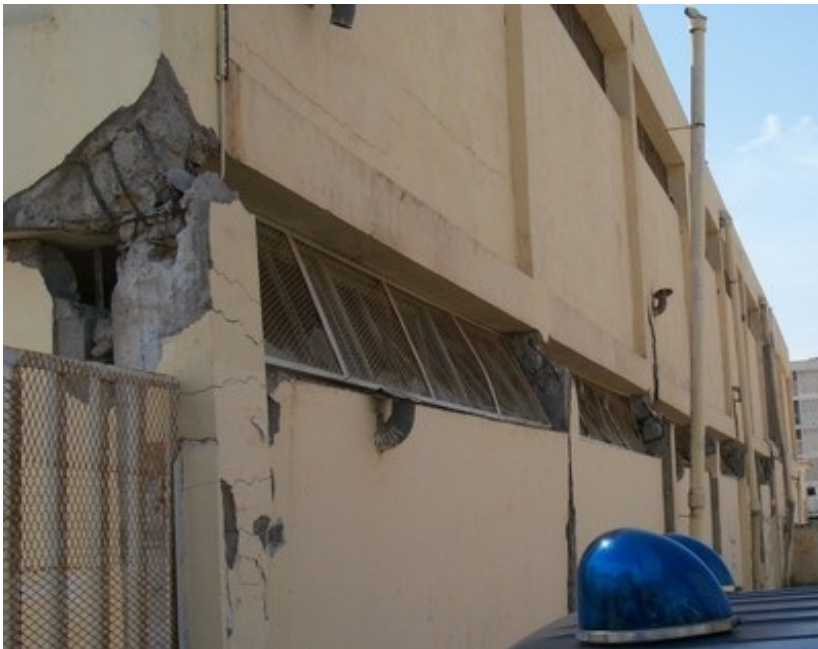
Captive columns in a reinforced concrete building damaged in the 2003 Boumerdes, Algeria earthquake (M. Farsi)
