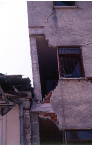
Pounding damage in adjacent buildings of different heights affected by the 1999 Turkey earthquakes (Gulat, Ascheim, and Spence, World Housing Encyclopedia Report 64 )
