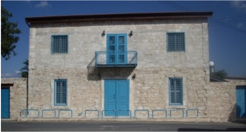
A two-storey sandstone masonry building, West Cyprus (A. Pomonis)
