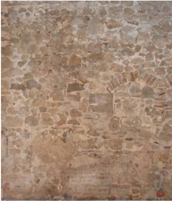
Heterogeneous (mixed) masonry wall uses a combination of limestone and limestone, as well as clay bricks for arching lintels, L'Aquila, Italy (A. Benedetti)
