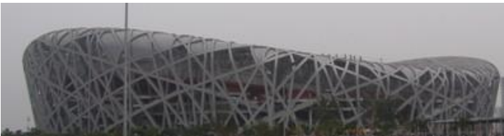
Birds Nest Stadium in Beijing, China has a 3-D braced frame structural system (S. Brzev)
