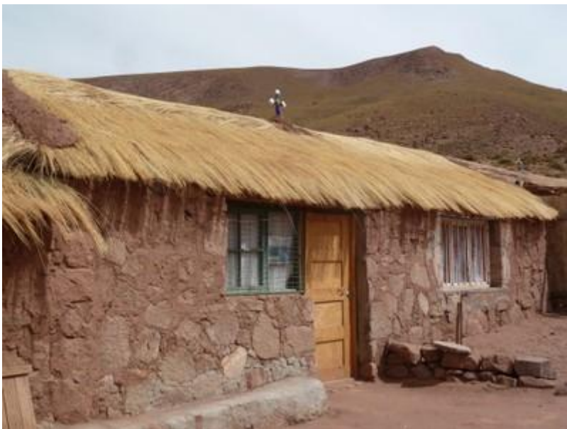
Semi-dressed stone masonry in mud mortar, Chile (S. Mihaldzic)
