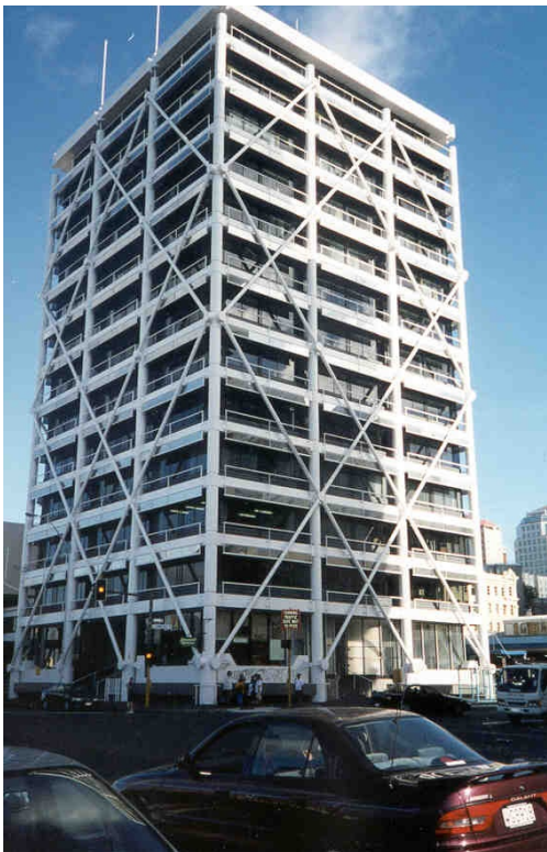
Energy dissipation devices were installed in the Union House, Auckland, New Zealand (S. Brzev)
