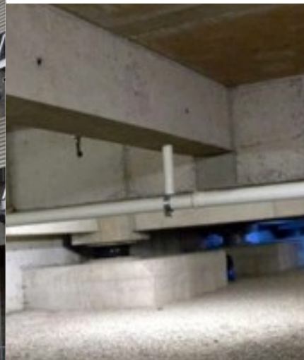
Edificio San Agustín (Catholic University of Chile) is concrete building in Santiago, Chile built in 2001 and equipped with lead core base isolation devices; the left photo shows the building and the right photo shows a typical isolation device located in the basement (S. Brzev)
