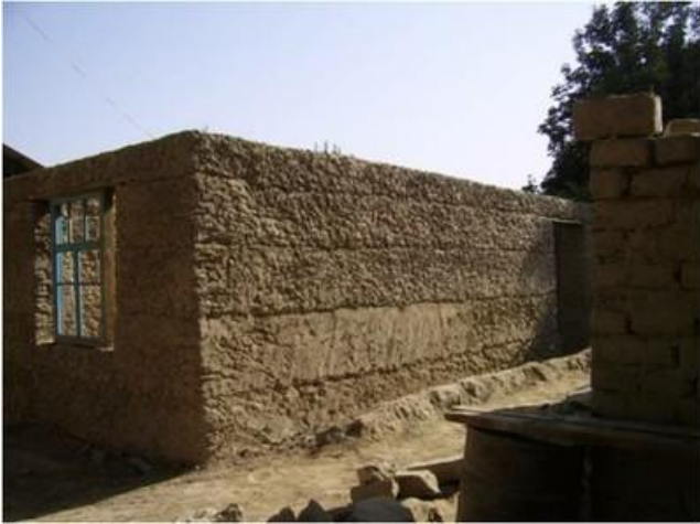
Rammed earth construction, Tajikistan (J. Niyazov)
