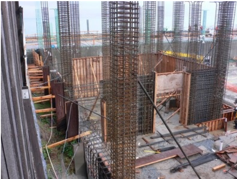
Cast-in-place construction (columns), California (A. Charleson)
