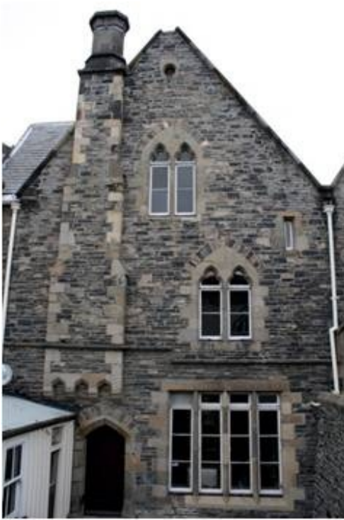
A 19th century stone masonry construction: exterior wall wythe is fine grained grey Halswell basalt, with facing stones and base course of pinkish-brown Port Hills trachyte and string courses of speckled Hoon Hay basalt; Canterbury Provincial Buildings complex, Christchurch, New Zealand (W. Clark)
