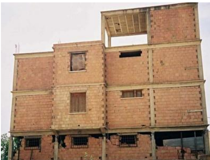
This reinforced concrete frame building with hollow clay tile infills in Algiers was under construction at the time of the 2003 Boumerdes, Algeria earthquake, and it suffered damage at the first storey level (S. Brzev)
