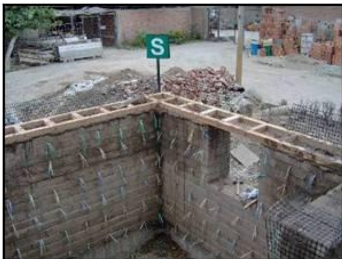
Adobe building with a wood bond beam at eaves level, Peru (M. Blondet)
