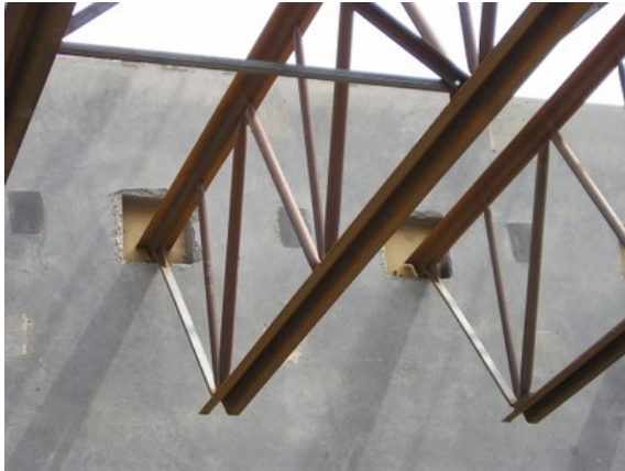
Steel trusses (Open Web Steel Joists) supported by precast concrete tilt-up walls, Canada (S. Brzev)
