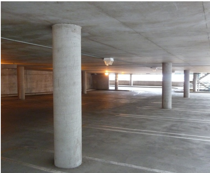
Flat plate concrete construction, parking garage, USA (S. Brzez)
