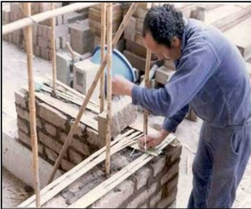
Adobe wall with vertical cane reinforcement, Peru (M. Blondet)
