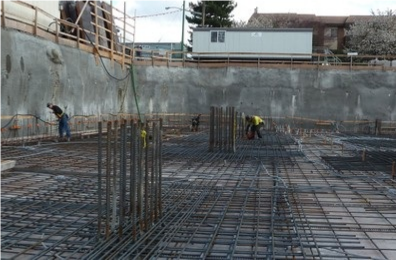
Reinforced concrete slab and columns under construction, Canada (S. Brzev)
