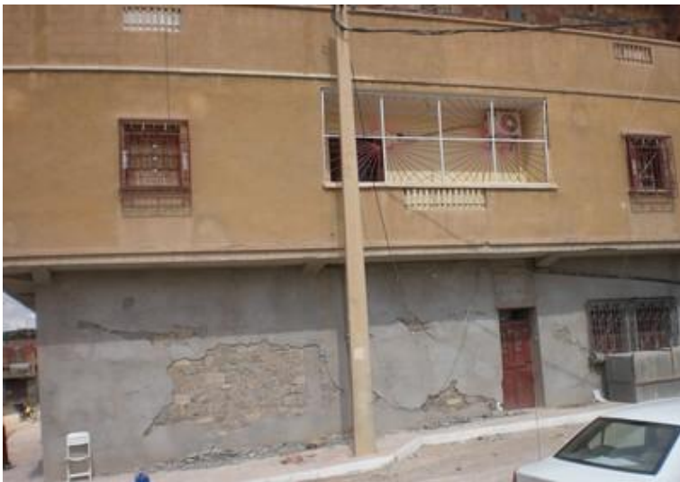
Reinforced concrete frame infilled with stone masonry panels in M'Sila damaged in the 2010 Algeria earthquake (M. Farsi)
