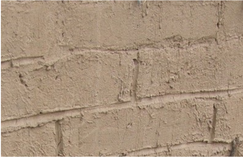
Mud mortar and adobe blocks, Peru (S. Brzev)
