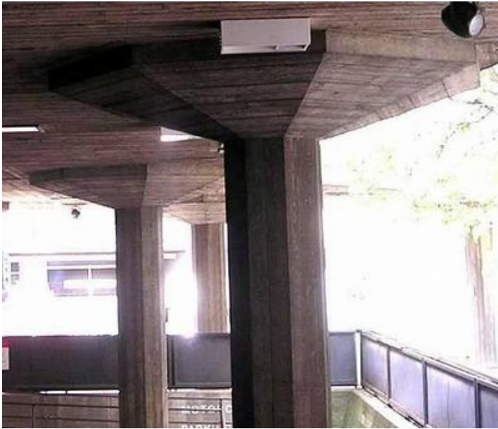
Reinforced concrete flat slab with a column capital, London, UK (S. Brzev)
