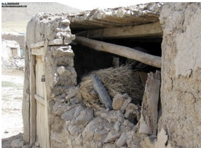
Flat wooden roof with heavy mud and straw overlay, Iran (A. Mahdizadeh, M. Yekrangnia)
