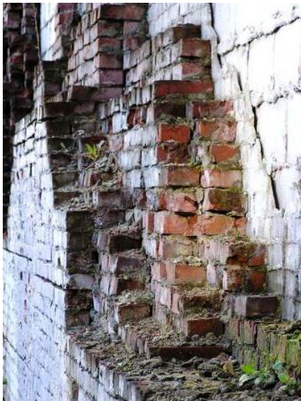
An older partially demolished multi-wythe brick masonry wall in Vancouver, Canada (B. McEwen)
