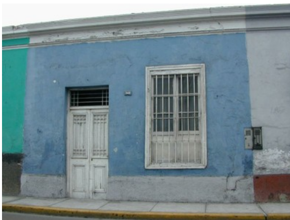
Adobe masonry walls overlaid by plaster, Peru (C. Loaiza and M. Blondet, World Housing Encyclopedia Report 52)
