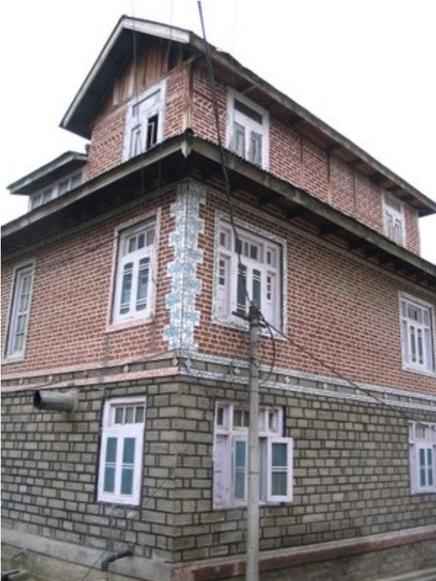
A hybrid building with stone masonry wall at the ground floor, brick masonry wall at the second floor, and Dhajji Dewari construction (note wooden posts) at the top floor level, Kashmir, India (D. Rai)
