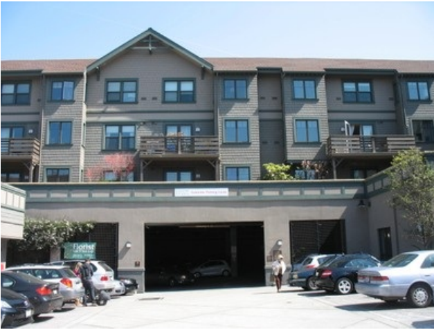
Reinforced concrete frames at the ground floor level and wood frame apartments above - ground floor usually used for parking, California (D. Bonowitz). A building with precast reinforced concrete frame at the ground floor level and wood frame above collapsed in the 1994 Northridge, California earthquake (the concrete frame collapsed and the building lost ground floor) (FEMA 454)
