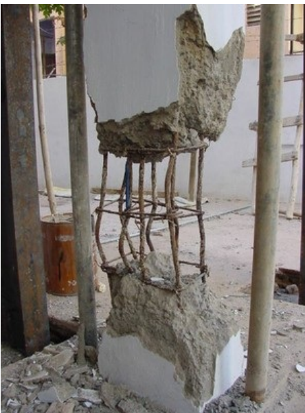
Failure of reinforced concrete columns at the ground floor level of a building with the soft storey irregularity in the 2001 Bhuj, India earthquake; the columns were characterized by non-ductile details, such as widely spaced ties and 90 degree hooks in ties (C.V.R. Murty, EERI)
