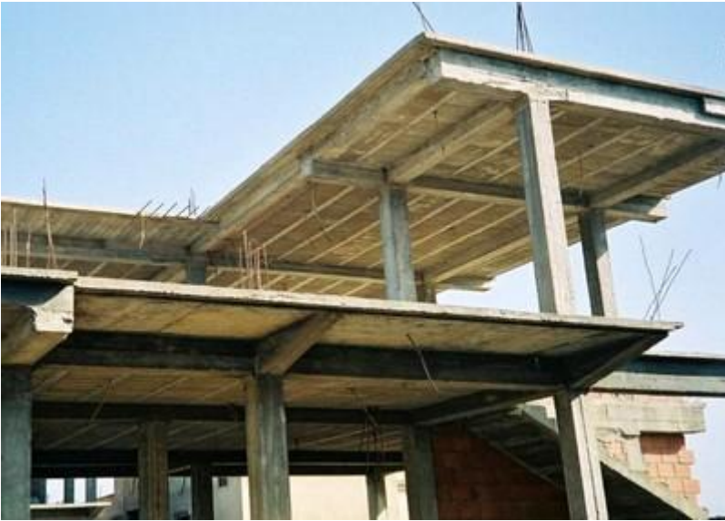
Floor system consisting of concrete masonry units and reinforced concrete joists cast in-situ, Algeria (S. Brzev)
