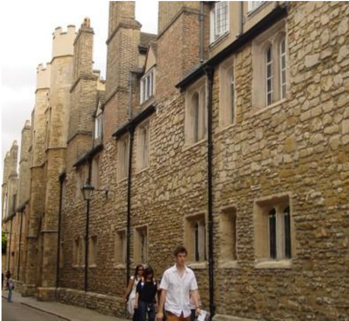
Random rubble stone masonry, Cambridge, United Kingdom (S. Brzev)
