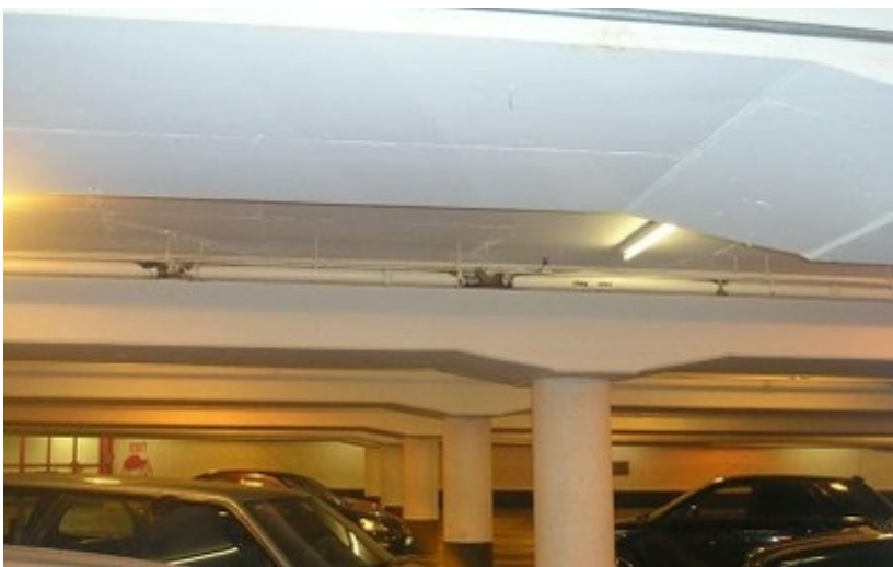
Reinforced concrete slab supported by beams, Canada (S. Brzev)
