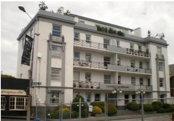
Pre-1976 in-situ reinforced concrete wall construction, Christchurch, New Zealand (J. Bothara)
