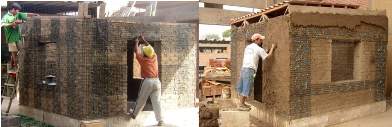
Adobe walls reinforced with polymer mesh, construction phase; note the mesh overlaid with mud plaster on the right photo (N. Tarque)
