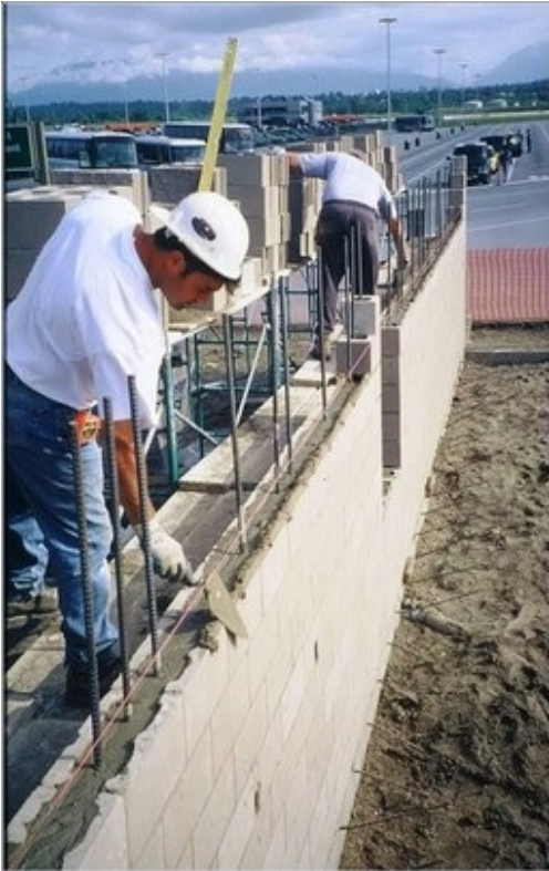
Reinforced masonry construction using concrete block masonry and steel reinforcement, Canada (left: B. McEwen; right: Anderson and Brzev, 2009)
