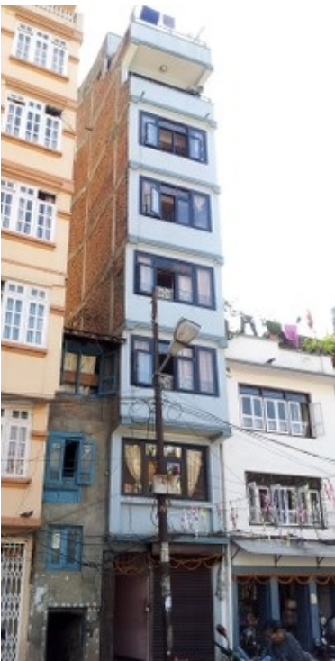
Adjacent buildings of different height, pounding potential, Kathmandu, Nepal (K. Porter)
