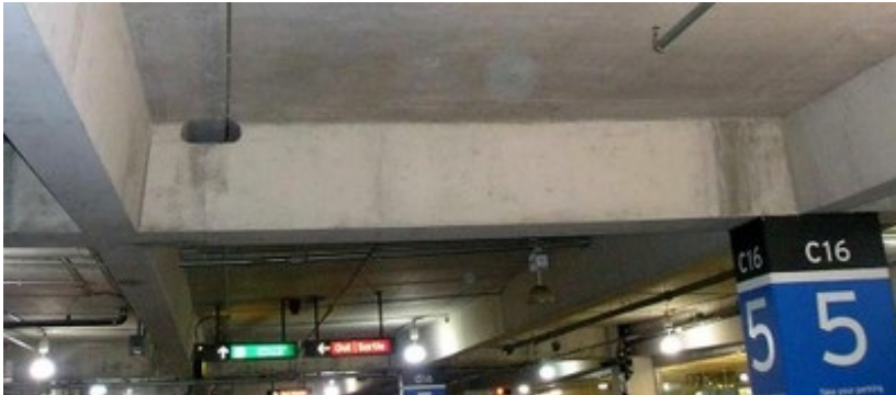
Reinforced concrete slab supported by beams, Canada (S. Brzev)
