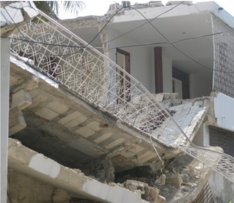
Floor slab system consisting of cast-in-place reinforced concrete voided with concrete blocks was observed in Haiti after the 2010 earthquake (top photo - A. Irfanoglu and bottom photo - A. Lang)
