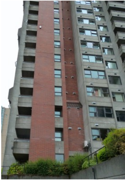
An example of a masonry veneer in a reinforced concrete building in Vancouver, Canada; veneer can be identified by weep holes, as shown in the photo (S. Brzev)
