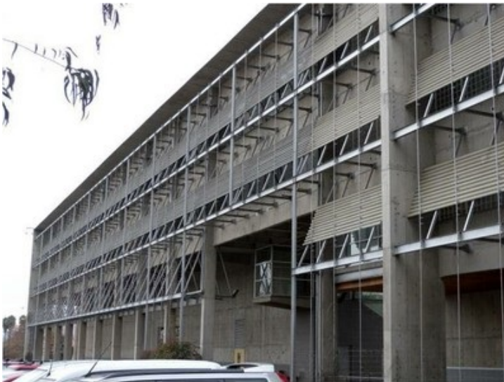
Edificio Comunidad Andalucía, a four-storey masonry building in Santiago, Chile was built in 1992 and it is equipped with the high damping rubber isolation devices; an exterior view of the building is shown left (S. Brzev) and a floor plan showing isolator locations is shown right (M. Moroni)
