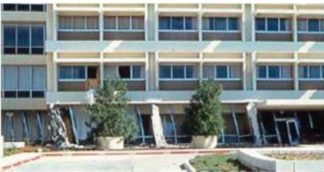
Olive View Hospital suffered severe damage in the 1971 San Fernando, California, due to discontinuous reinforced concrete shear walls shown shaded on the vertical section drawing. A soft two-storey layer of rigid reinforced concrete frames supported a stiff shear wall-frame structure above. Severe damage occurred in the soft storey portion, as shown in the photo (FEMA 454)
