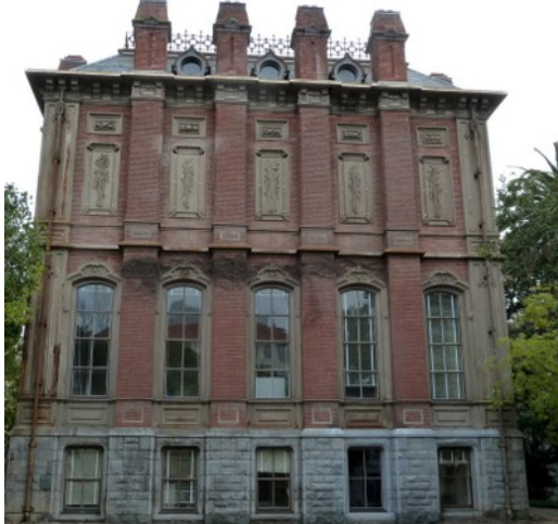
Stone masonry at the ground floor level and brick masonry above, Berkeley, California (S. Brzev)
