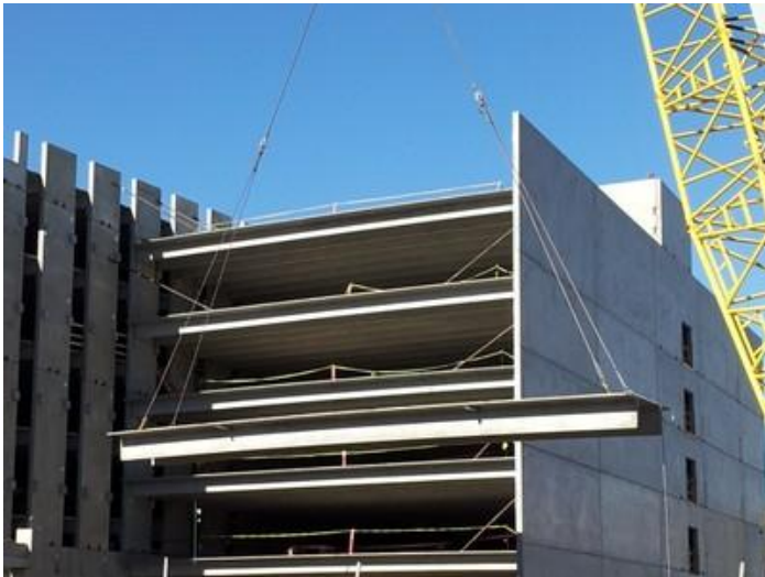
Double-tee beam lifted by crane at the construction site, Denver, USA (K. Porter)
