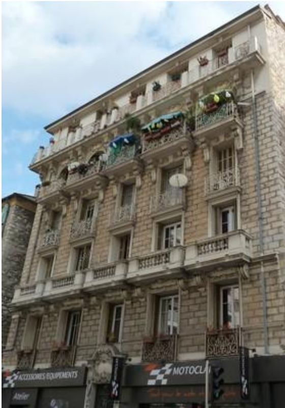
Limestone masonry walls in a six-storey residential building, Nice, France (S. Brzev)
