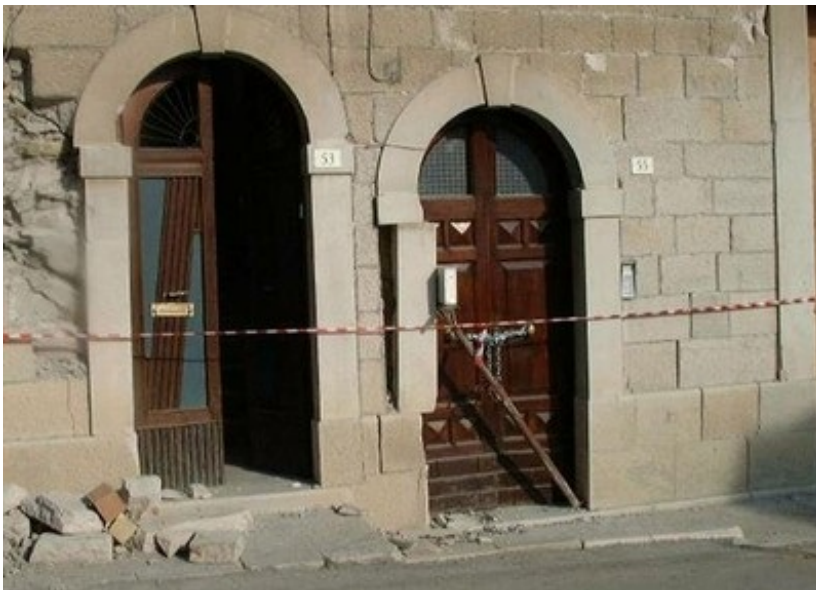
A stone masonry wall (exterior wall) built using tuff stone in San Giuliano damaged in the 2002 Molise earthquake, Italy (A. Benedetti)
