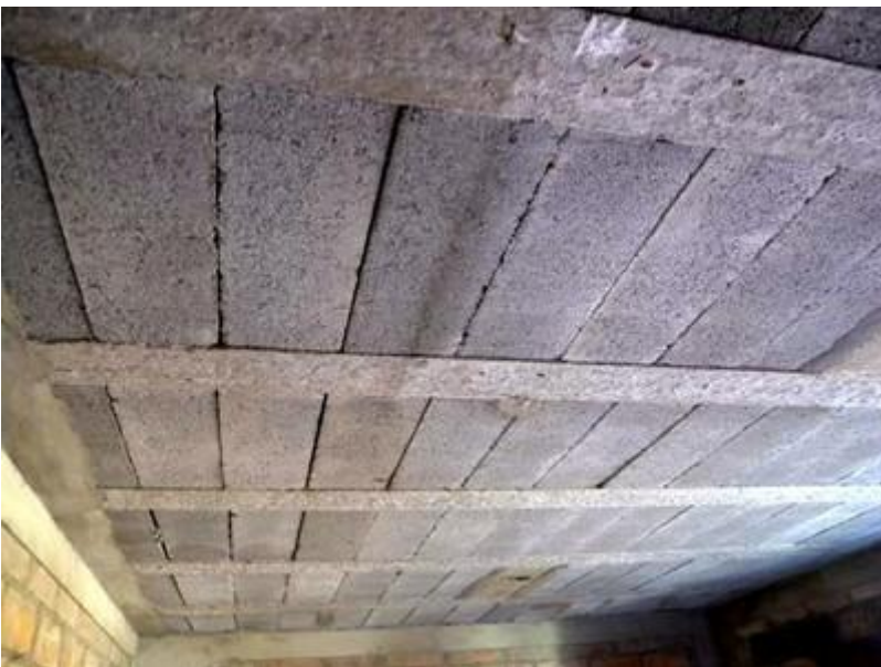
Floor system consisting of concrete masonry units and cast-in-situ reinforced concrete joists (known as "Tralix" system), Chile (S. Brzev)
