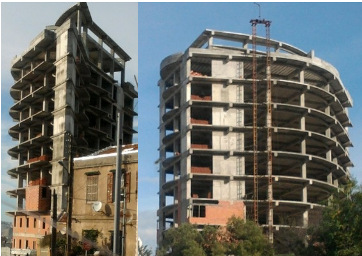
Dual frame-wall system is common for contemporary reinforced concrete building construction in Algeria (M. Farsi)
