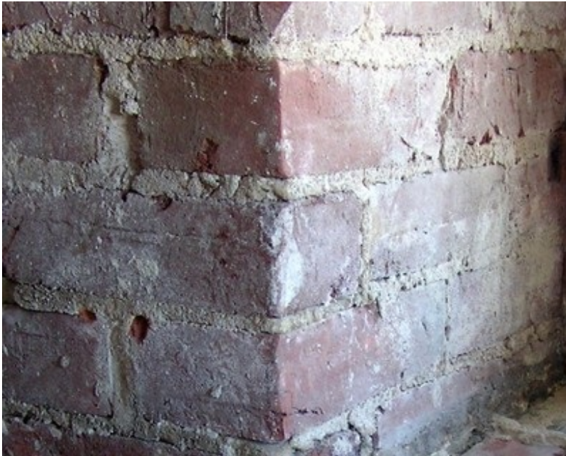
Fired clay brick masonry in lime mortar, Canada (Ojdrovic Engineering)
