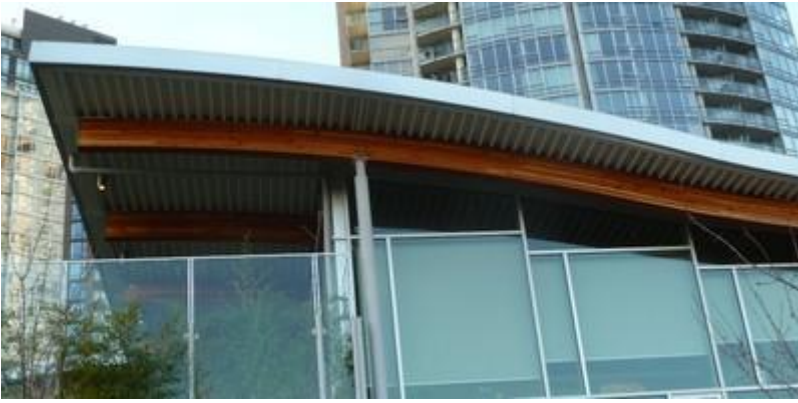
Curved wooden glulam beams supporting light metal roof covering, Canada (S. Brzev)
