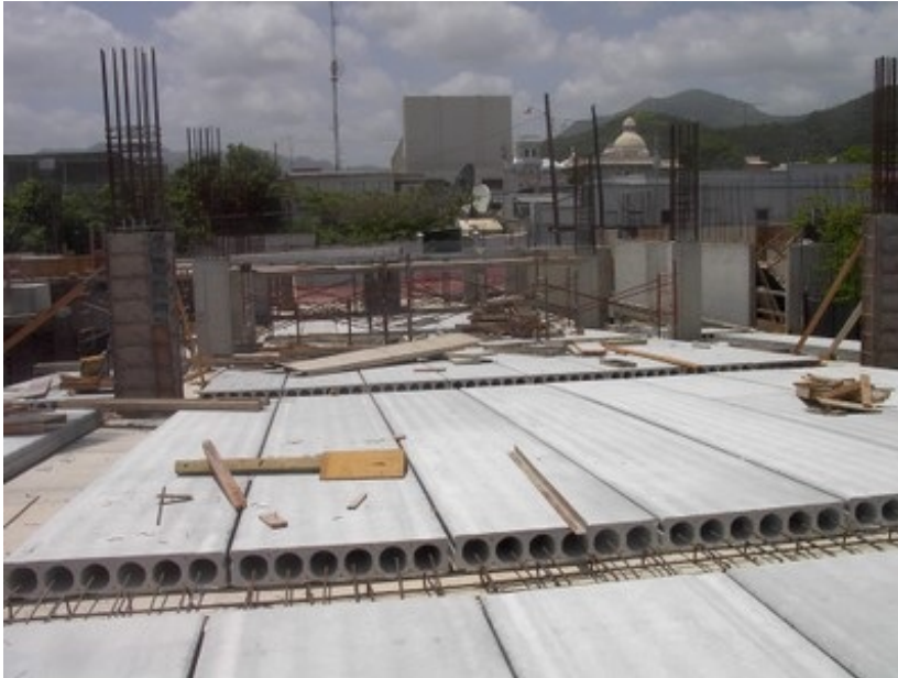
Precast concrete hollow core slabs ( tropicalconcrete.com )
