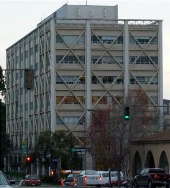
Exterior steel braced frame as a retrofit solution, University Hall, University of Berkeley, California (S. Brzev)
