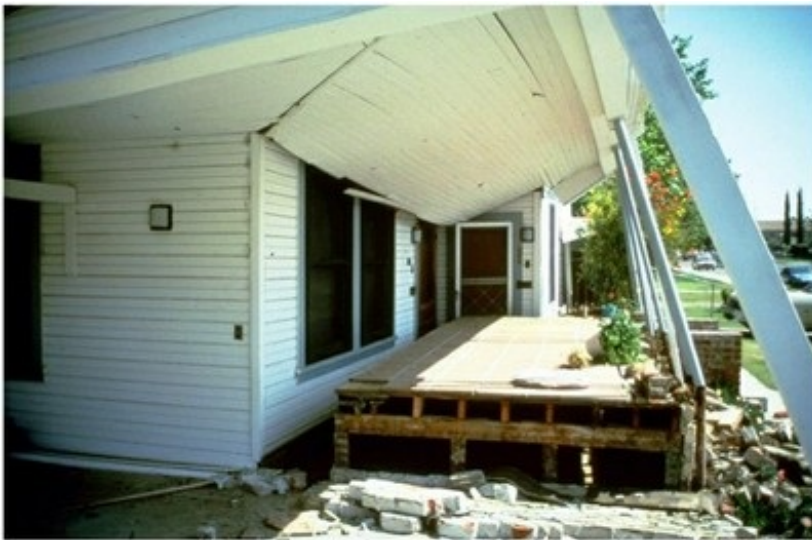
Collapse of a wood-frame house which slid over the cripple wall, 1983 Coalinga, California earthquake (EERI)
