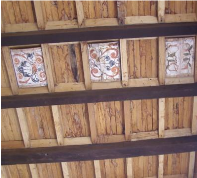
Wooden beam and joist roof, Peru (S. Brzev)
