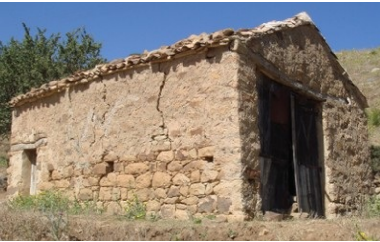
Sandstone masonry walls in Ben-Daoud damaged in the 2010 earthquake, Algeria (M. Farsi)
