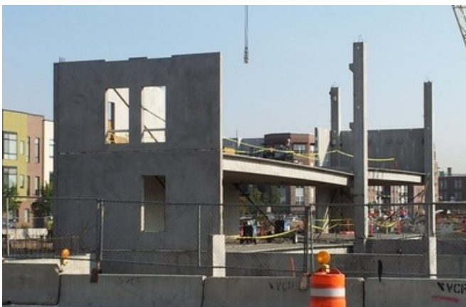
Erection of precast concrete wall panels, New Zealand (A. Charleson)
