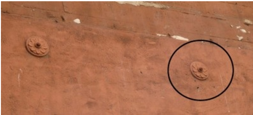
A typical wall anchor, consisting of a steel rod and an exterior steel plate exposed at the exterior; note that anchor plates are of different shapes and sizes (S. Brzev)
