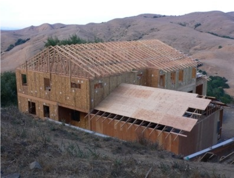
Wood-based sheets on rafters or purlins, California (A. Charleson)
