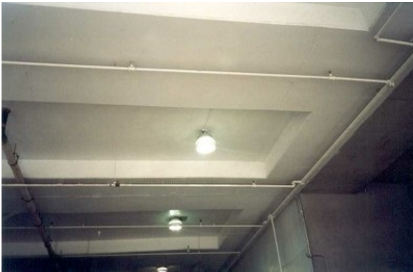
Reinforced concrete slab band system, Canada (S. Brzev)
