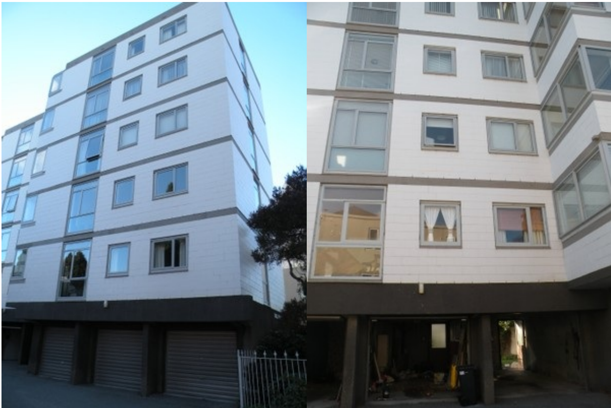
A six-storey building damaged in the February 2011 Christchurch, New Zealand earthquake has reinforced concrete walls at the ground floor level and reinforced masonry construction above (in the form of interior reinforced concrete block walls in the interior and cavity walls at the exterior) (J. Centeno)
