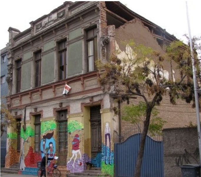
Unreinforced brick masonry damaged in the 2010 Maule, Chile earthquake (S. Brzev)
