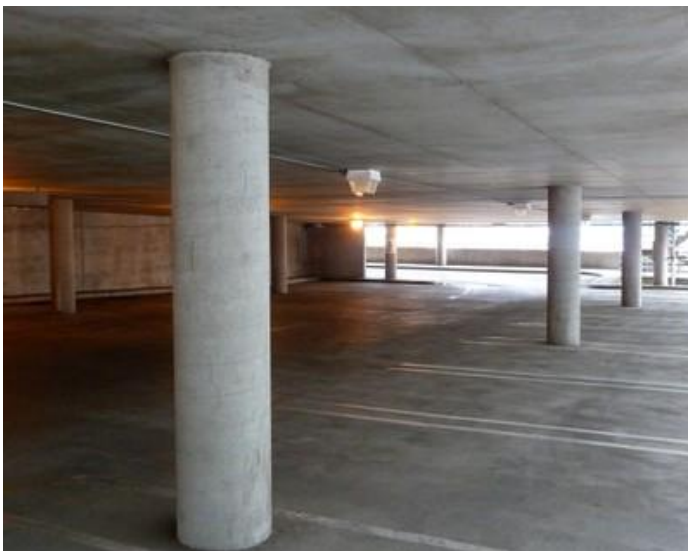
Reinforced concrete flat plate system, Eugene, USA (S. Brzez)
