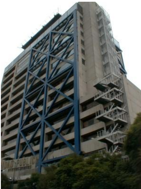
Exterior braced frame as a retrofit scheme for a reinforced concrete building, Mexico (C. Scawthorn)
