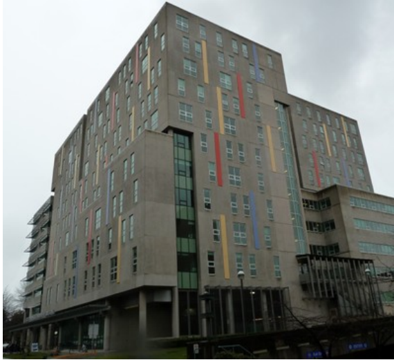
Cast in-place reinforced concrete exterior walls, Vancouver, Canada (S. Brzev)
