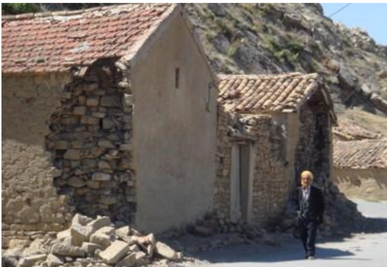
Limestone masonry wall in Ben-Daoud damaged in the 2010 Algeria earthquake (M. Farsi)
