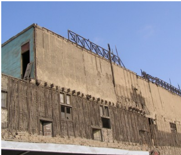
Mud walls reinforced with bamboo reinforcement, Kenya (K. Jaiswal)
