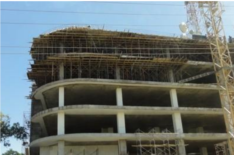
A reinforced concrete building with flat plate system under construction, Kenya (K. Jaiswal)
