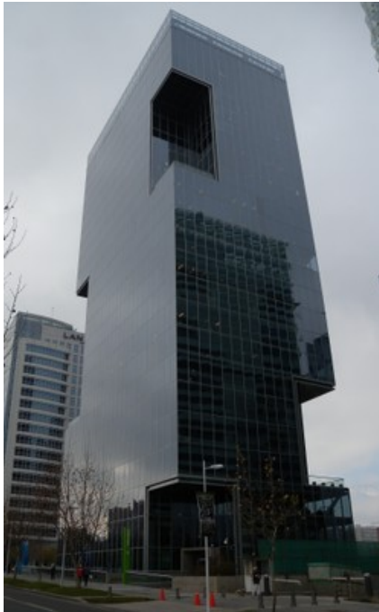
A highrise office building with glass curtain walls, Santiago, Chile (S. Brzev)
