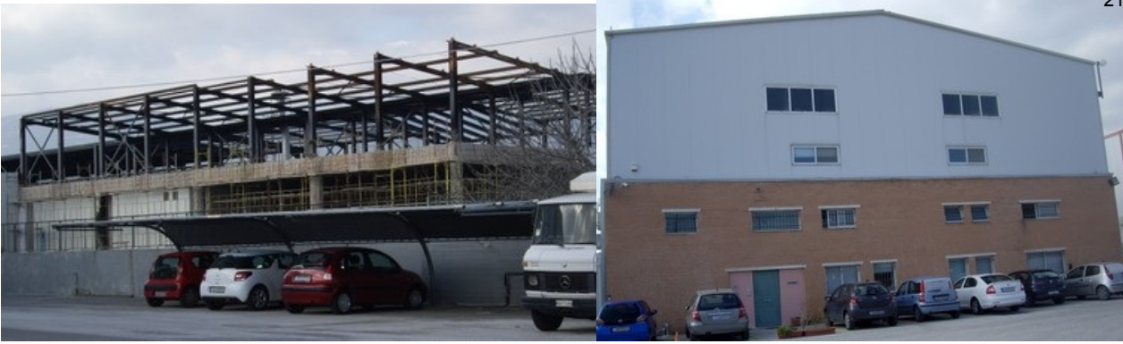
An example of a hybrid system with reinforced concrete frame at the ground floor level and steel frame above, Athens, Greece (the left photo shows a building under construction and the right photo shows a similar building when completed) (A. Pomonis)
