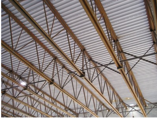
Steel trusses (open web steel joists) supporting composite steel and concrete floor system, Canada (S. Brzev)
