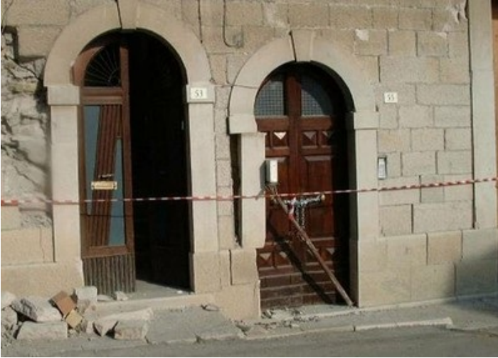
A wall built using dressed tuff stone exterior wythe over a rubble masonry in San Giuliano damaged in the 2002 Molise earthquake, Italy (A. Benedetti)
