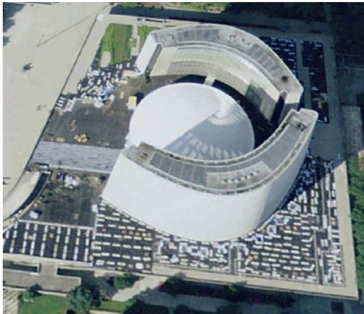
City Hall in Toronto, Canada has two half-circle office towers, curving around a circular council chamber; the towers can be classified as U-shaped building plans (Map data ©2013 Google, DigitalGlobe)
