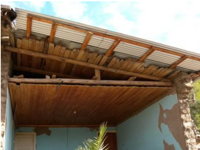
Wooden structure supporting wooden planks and steel sheet roofing, Chile (S. Brzev)
