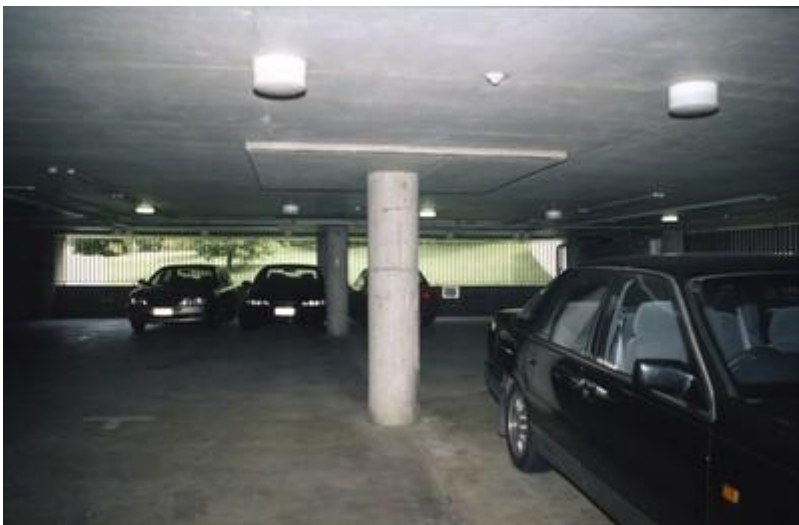
Flat slab, Australia - note drop panels beneath the slab (A. Charleson)
