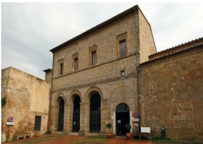
Tuff stone was used for the construction of Bourbon del Monte Palace (16th century), Sovana, Italy ( www.fototoscana.it )
