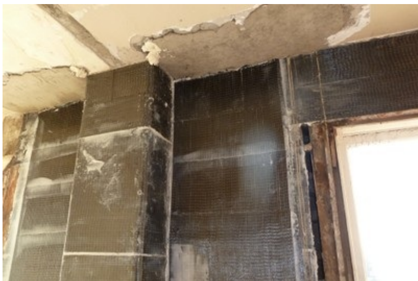
Reinforced concrete wall and column retrofitted with carbon fiber wrap, USA (S. Brzev)
