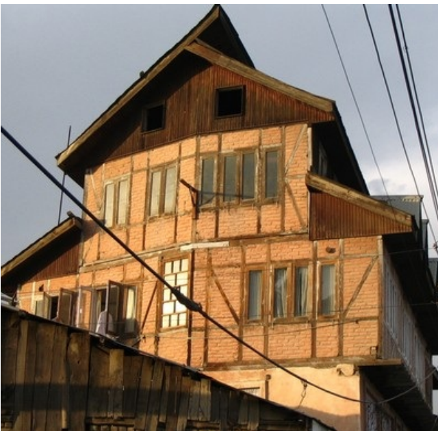
Wood-reinforced brick masonry known as Dhaji Dhewari in Kashmir, India (S. Brzev)
