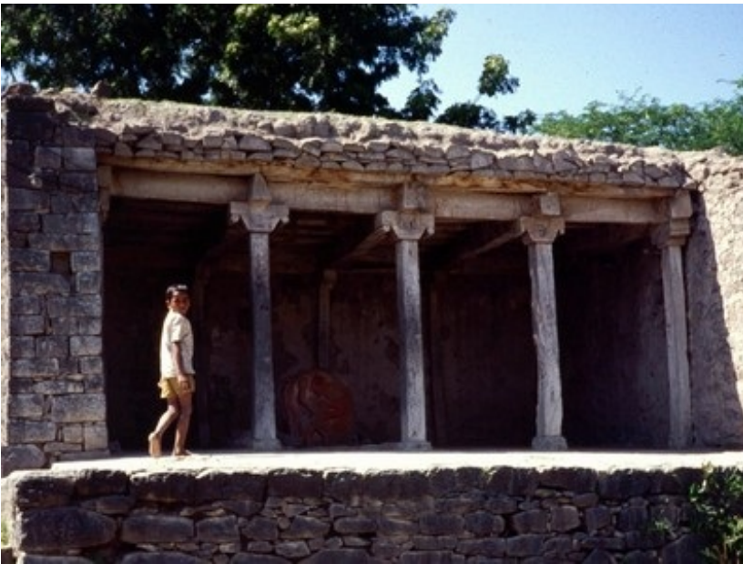
Flat wooden roof structure supporting heavy mud covering, India (S. Brzev)
