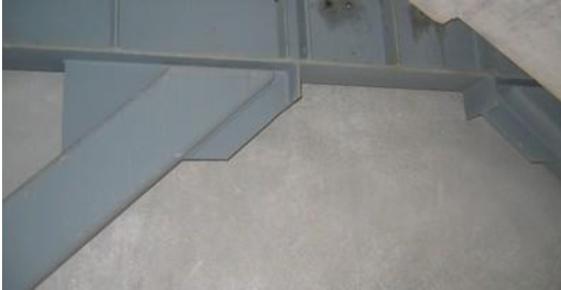
Welded connection of steel brace to gusset plate, New Zealand (A. Charleson)
