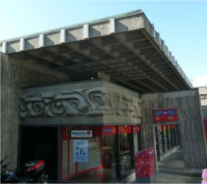
Flat concrete roof (w affle slab system), Vancouver, Canada (S. Brzev)
