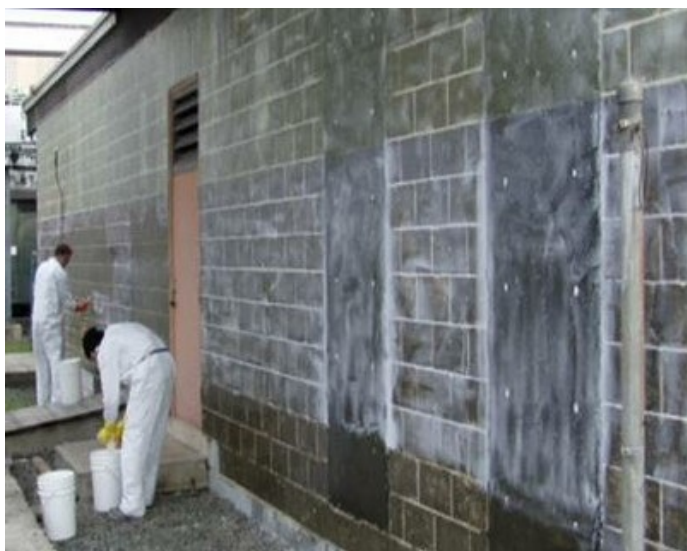
Concrete block masonry reinforced with fibre reinforced composite mesh, Canada (J. Sherstobitoff)
