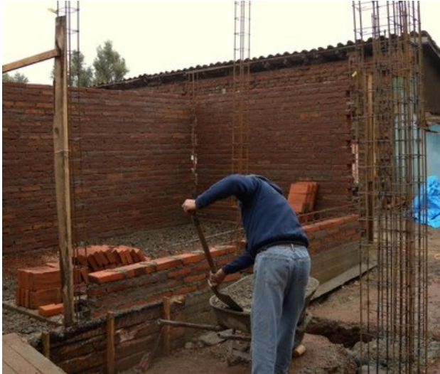
Confined masonry wall under construction using clay brick units, Chile (S. Brzev)
