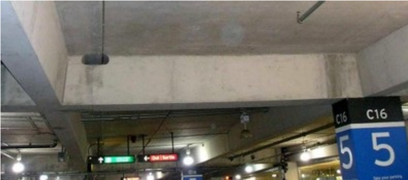
Reinforced concrete slab supported by beams, parking garage, Canada (S. Brzev)
