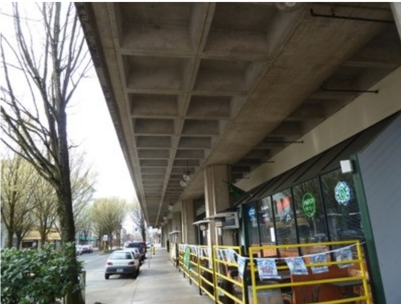
Reinforced concrete waffle slab with beams, USA (S. Brzev)
