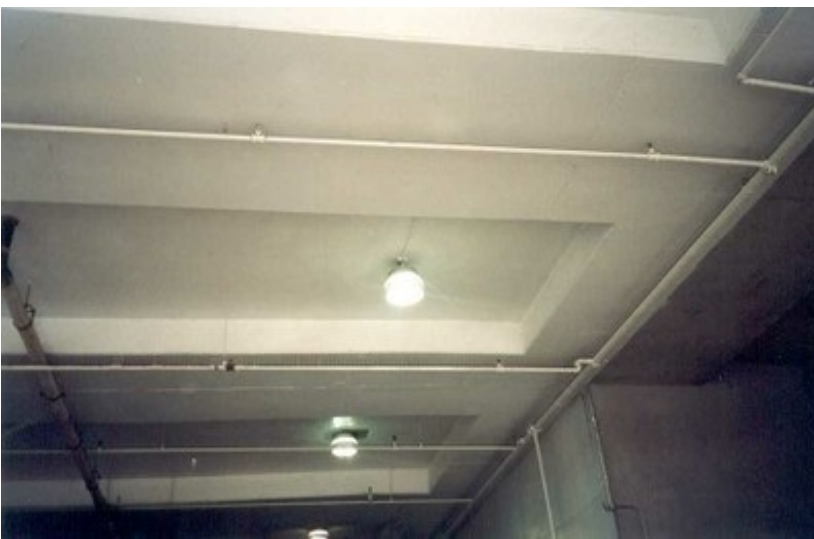
Reinforced concrete slab band floor system in a parking garage, Canada (S. Brzev)
