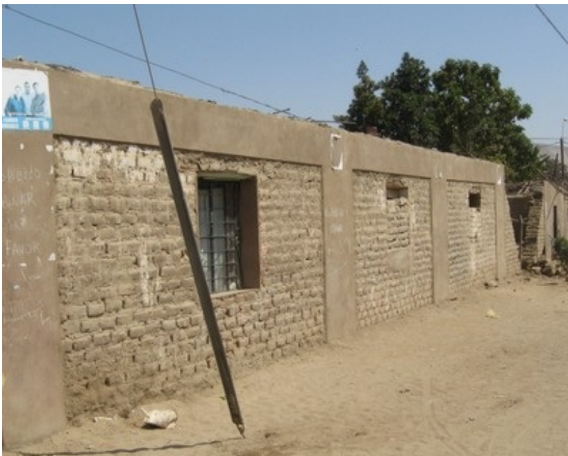
An adobe building reinforced externally with steel wire mesh overlaid with cement plaster, Peru (N. Tarque)
