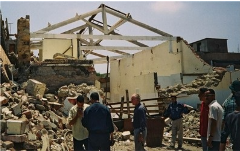
Unreinforced masonry buildings often show non-ductile performance and suffer damage in major earthquakes, such as the 2003 Boumerdes, Algeria earthquake (S. Brzev)
