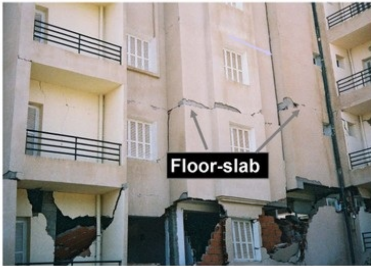
Two adjacent reinforced concrete buildings on a sloped ground suffered a major damage in the 2003 Boumerdes, Algeria earthquake; the buildings had an inadequate seismic gap, and the pounding effect was significant due to floor slabs at different elevations (S. Brzev)
