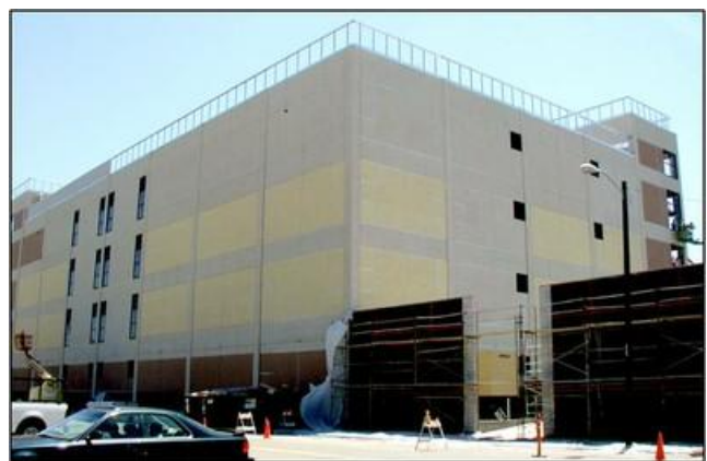
A cast-in-place reinforced concrete building with a Wall lateral load-resisting system, Oakland, California, USA (C. Scawthorn)
