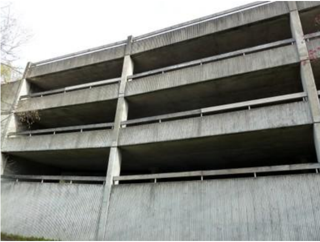
Reinforced concrete parking garage with flat slab system, USA (S. Brzev)
