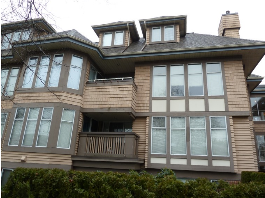
Wood plank cladding (lower level) and wood shingles (upper level), Canada (S. Brzev)
