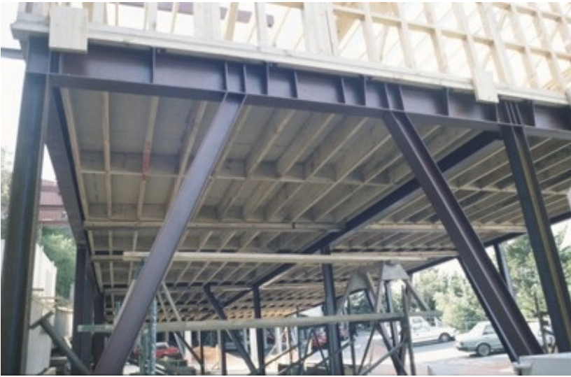
Wood based sheets on joists or beams, Wellington, New Zealand (A. Charleson)
