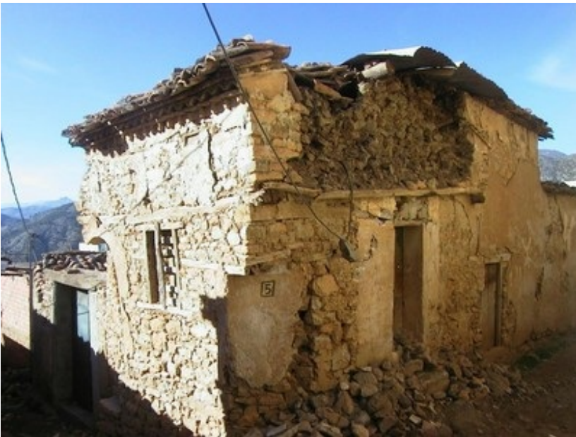
Sandstone masonry walls with timber reinforcement in Beni-Ourtlane damaged in the 2000 earthquake (M. Farsi)
