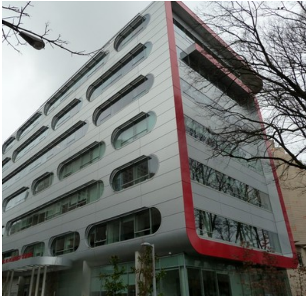
A building with exterior walls made of aluminum sheets, Vancouver, Canada (S. Brzev)
