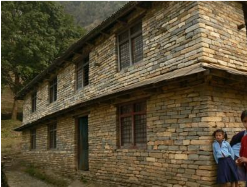
Limestone wall construction, school building, Nepal (M. Schildkamp)
