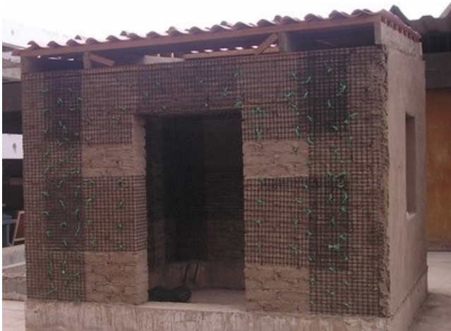
Adobe walls reinforced with polymer mesh, construction phase; note the mesh overlaid with mud plaster on the right photo (N. Tarque)
