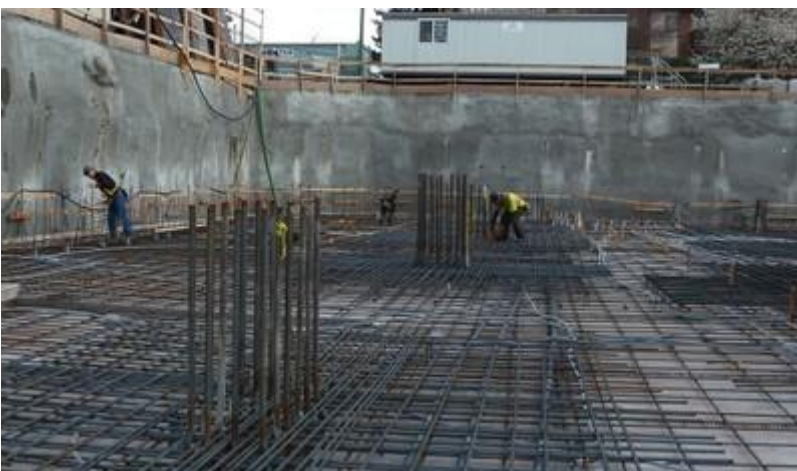
Reinforced concrete flat slab under construction, Canada (S. Brzev)
