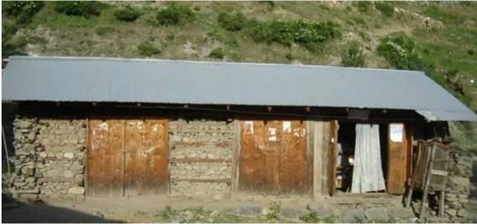
Rubble stone masonry in mud mortar with timber bands (local name: Bhatar), NWFP, Pakistan (J. Bothara)
