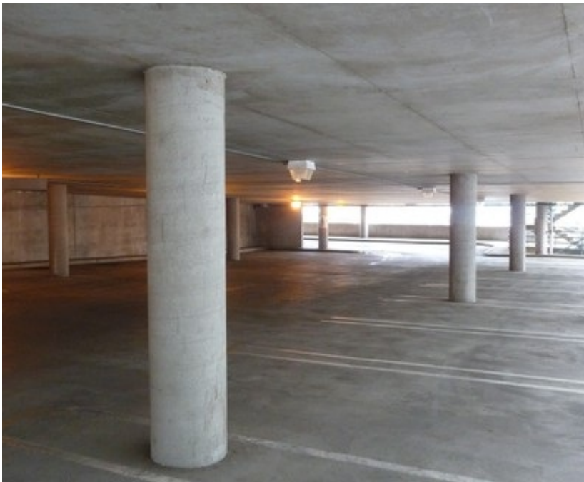
Reinforced concrete flat plate supported by columns, USA (S. Brzev)
