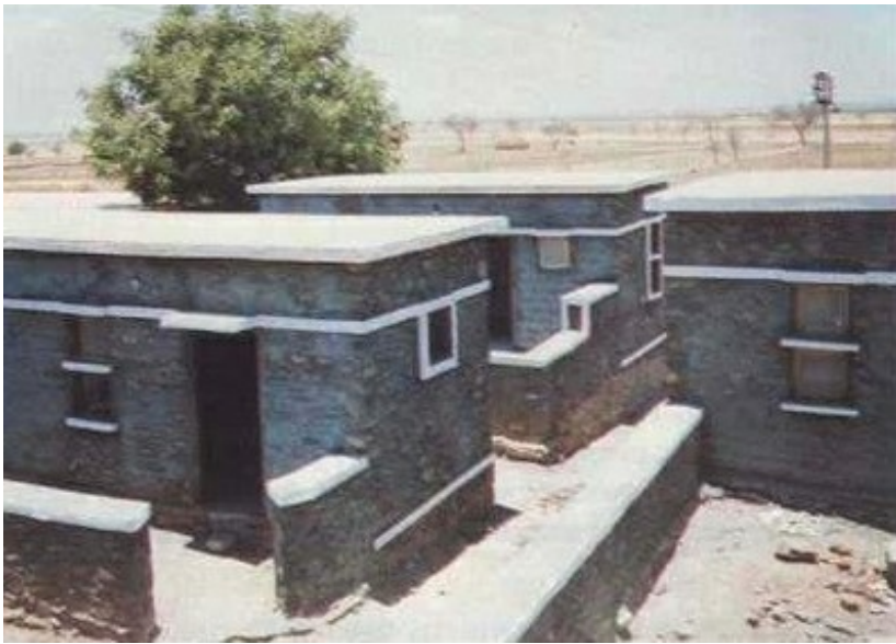
Stone masonry buildings with reinforced concrete bands at the lintel level, India (S. Brzev)
