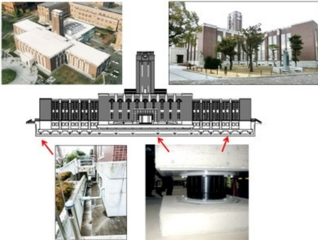
Kyoto University Clock Tower (Japan) is a 1925 concrete building retrofitted in 2000s using base isolation (drawing by M. Nakashima and photos by C. Scawthorn)
