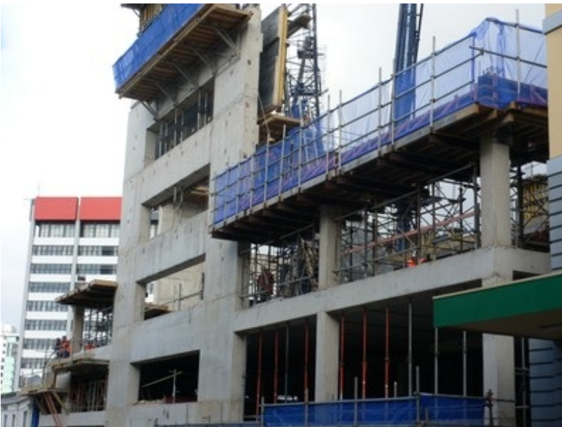
Reinforced concrete slab and columns under construction, Canada (S. Brzev)
