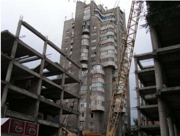
Reinforced concrete frame building under construction, Kyrgyzstan (U. Begaliev, A. Duishev, and R. Musakov)
