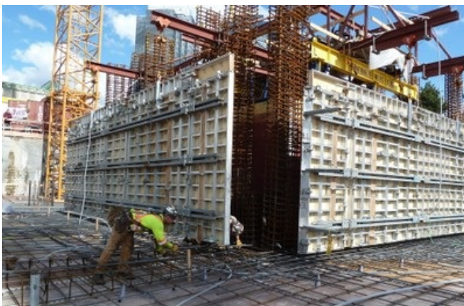
Cast-in-place concrete beam construction (note reinforcement and formwork), Canada (S. Brzev)
