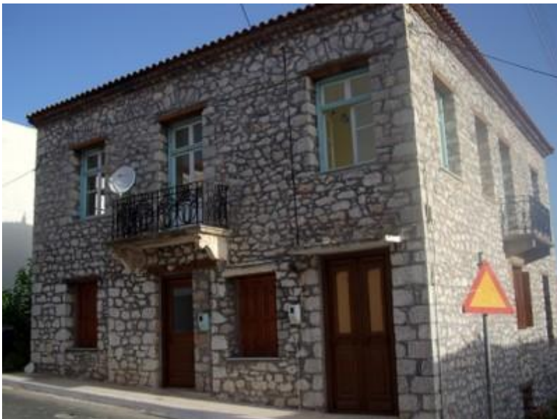
Loadbearing masonry walls built using limestone - note hewn stones in the corners and wooden lintels, Pylos, South West Peloponnese, Greece (A. Pomonis)
