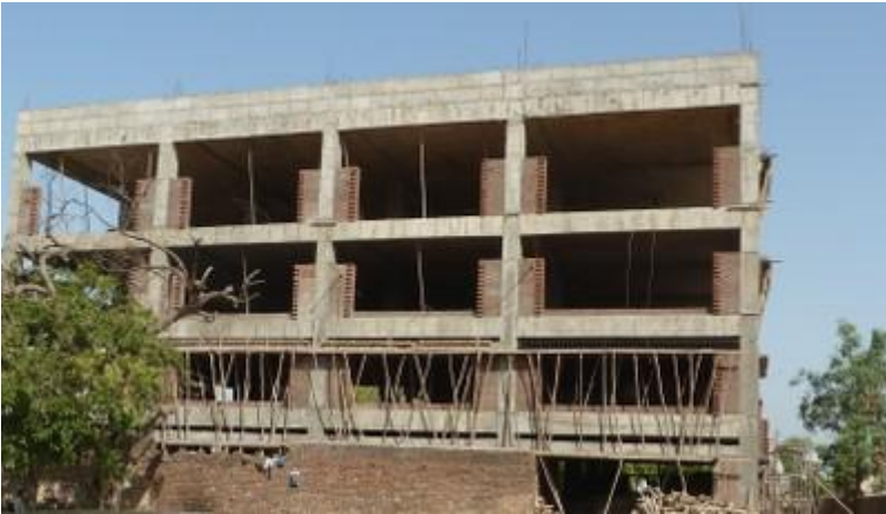
Reinforced concrete frame with brick masonry infills under construction, India (S. Brzev)
