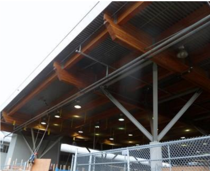
A roof structure consisting of steel decking supported by wooden glulam beams, Vancouver, Canada (S. Brzev)
