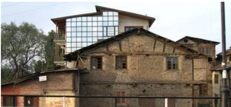
Taq is a timber-laced masonry construction where horizontal timbers are embedded in masonry walls at each floor level; this is a traditional construction found in Kashmir, India (D. Rai)
