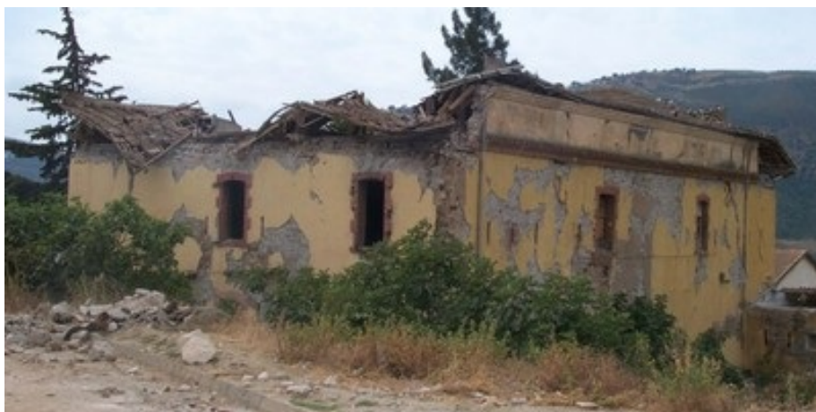
Unreinforced masonry building in Baghliia City experienced roof collapse in the 2003 Boumerdes, Algeria earthquake; the timber roof structure supported clay tile roof covering (M. Farsi)
