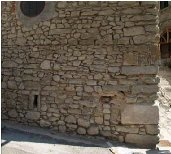
Rubble stone masonry, Italy (T. Schacher)
