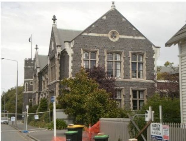
A stone masonry building built in 1920s in Christchurch, New Zealand; exterior stonework is Halswell basalt with Oamaru limestone facings (W. Clark)
