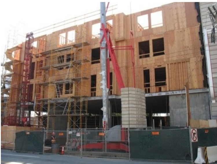
A hybrid system consisting of cast-in-place reinforced concrete frame construction at the ground floor level and wood frame construction above can be found in California (USA) and British Columbia (Canada) (D. Bonowitz)
