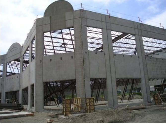
Tilt-up wall construction, Canada (S. Brzev)
