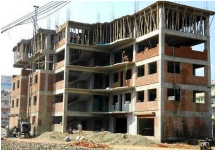
Reinforced concrete frame building with brick infill walls under construction, Kathmandu, Nepal (J. Bothara)
