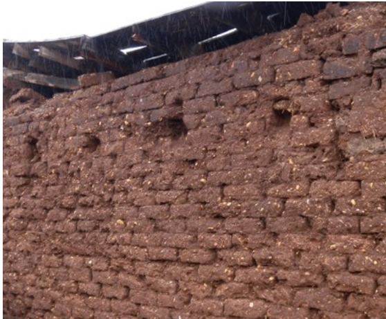
Adobe masonry walls: exposed (during construction), Chile (S.Brzev)
