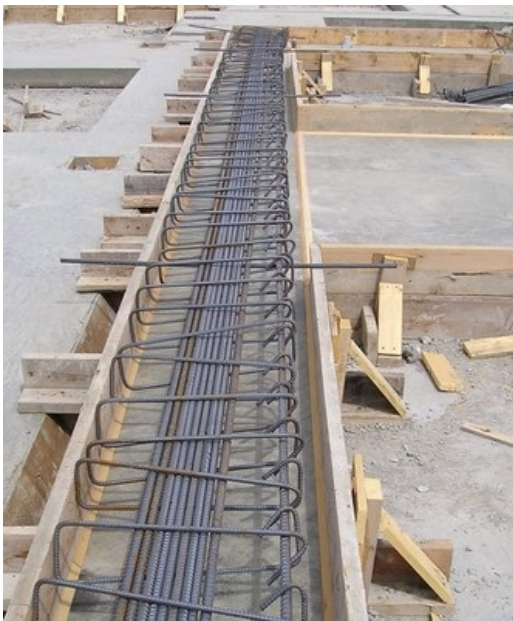
Cast-in-place concrete beam construction (note reinforcement and formwork), Canada (S. Brzev)
