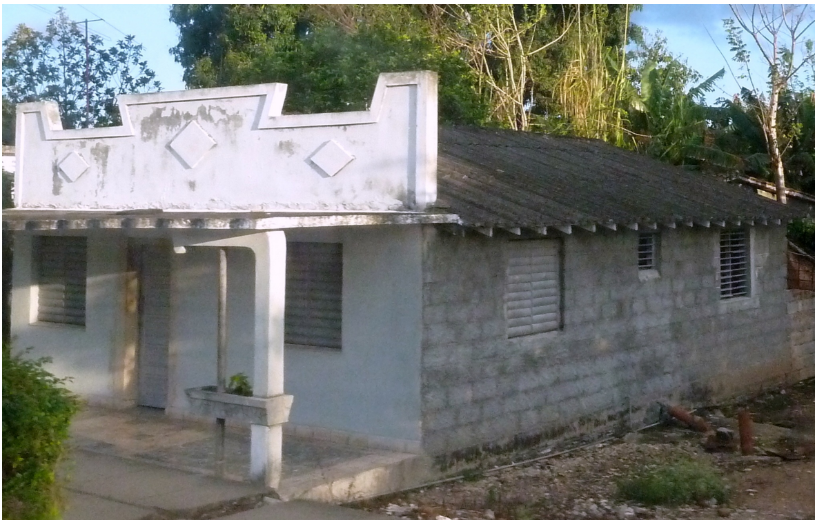
Concrete block construction, Cuba (S. Brzev)
