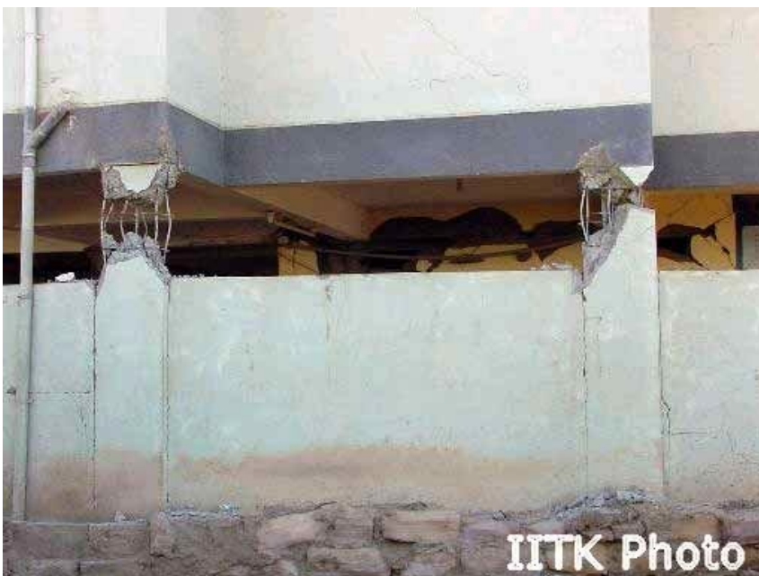
A building with captive columns suffered damage in the 2001 Bhuj, India earthquake (NICEE and IIT Kanpur)
