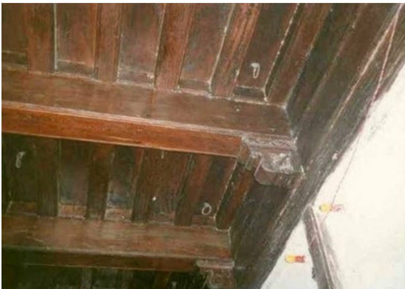
Wood floor with heavy overlay, India (S. Brzev)
