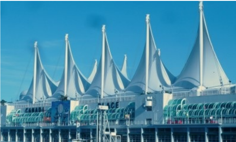
Canada Place in Vancouver, Canada, a tent-like structure that resembles a sailing ship, has a tensile membrane roof (S. Brzev)
