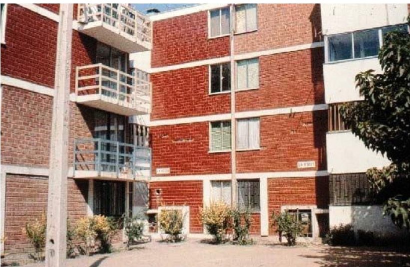
A hybrid system consisting of confined masonry at the bottom floor and reinforced clay block masonry above; this photo shows a building in Chile which suffered damage at the second floor in the 1985 Lolleo earthquake (M. Astroza)
