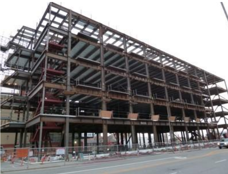
Steel building under construction, hot-rolled steel members, California (S. Brzez)
