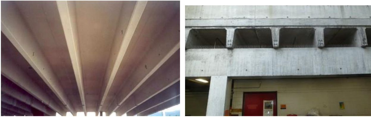
Precast concrete floor systems (double-tee units) are typically fabricated with a 50 mm flange and topped in the field with cast-in-place concrete (Canada, S. Brzev)
