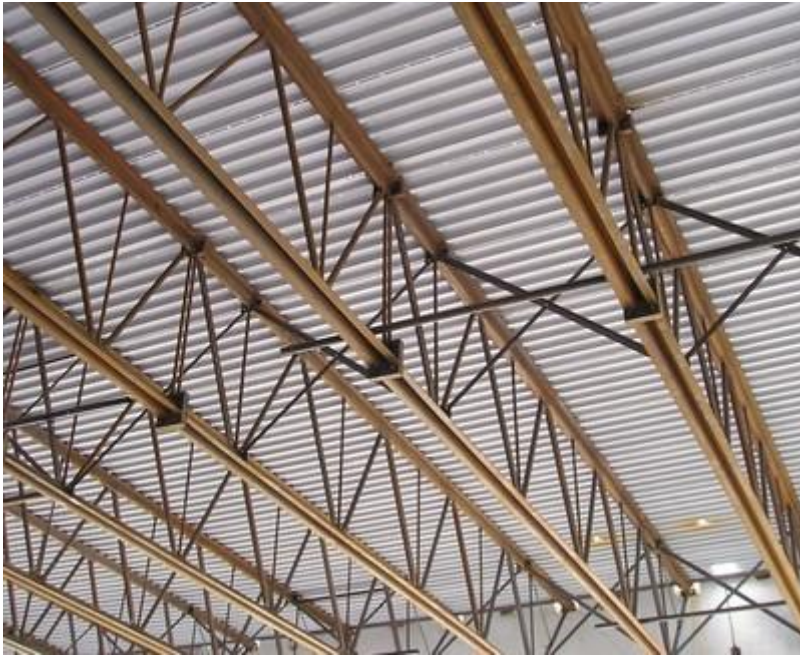
Detail of steel trusses (open web steel joists) supporting corrugated steel roofing, Canada (S. Brzev)
