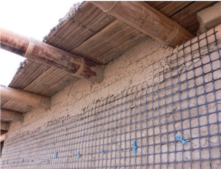
Adobe walls reinforced with a polymer mesh (geogrid) attached to the walls by plastic or nylon strings, Peru (N. Tarque)
