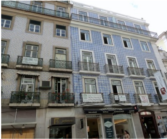
Many buildings in Lisbon, Portugal have glazed ceramic tiles bonded to exterior walls (S. Brzev)
