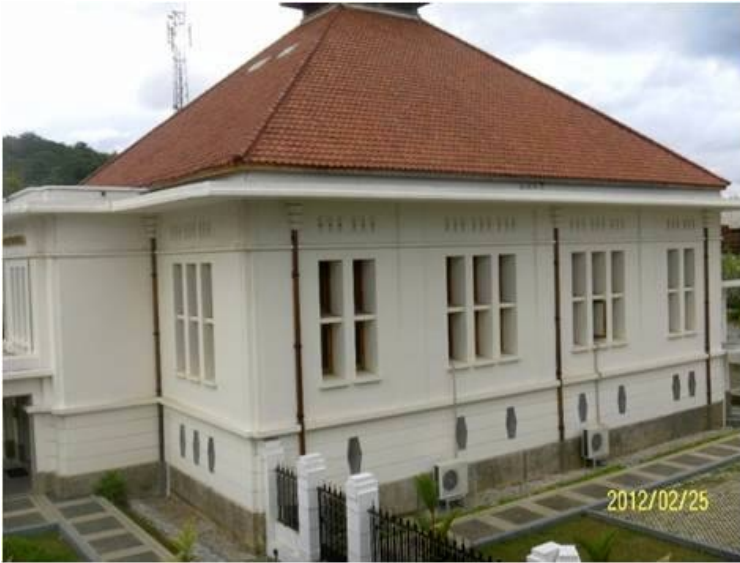
Unreinforced brick masonry construction (covered by plaster), Indonesia (J. Bothara)
