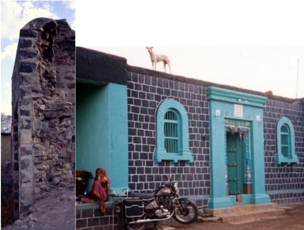
Semi-dressed stone masonry, Maharashtra, India (S. Brzev)
