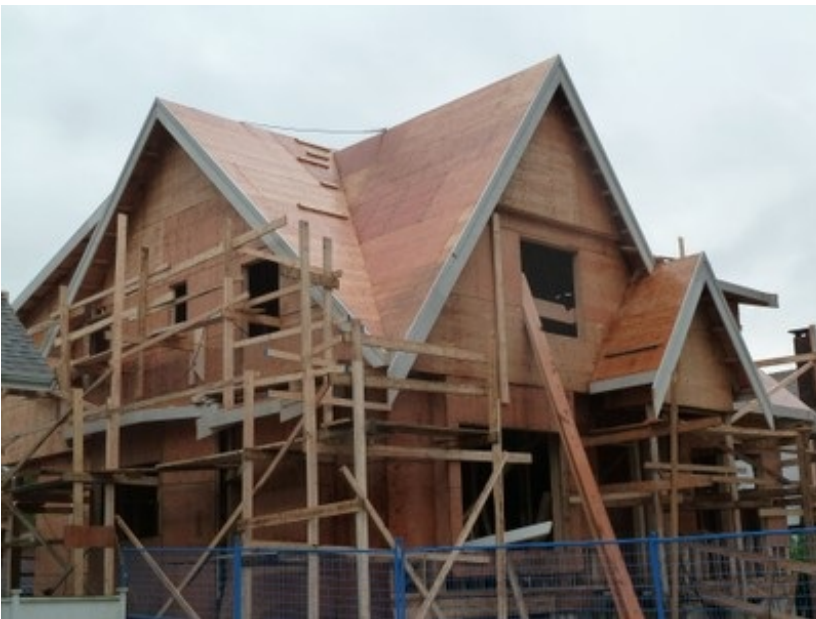
Plywood sheets over wood rafters or purlins - a roof under construction in Vancouver, Canada (S. Brzev)
