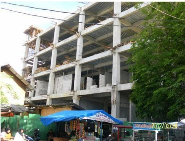
Reinforced concrete frame building with concrete block infill walls, Padang, Indonesia (J. Bothara)
