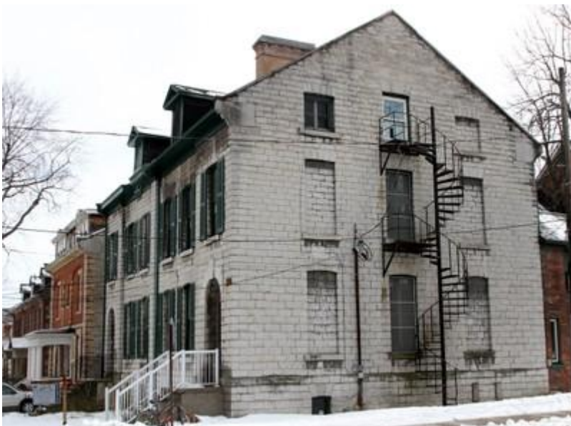
Limestone masonry, multi-family housing, Kingston, Ontario, Canada (J. Lee)
