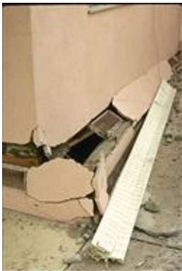
Cripple wall failure in the 1971 San Fernando, California earthquake (Courtesy of K.V. Steinbrugge and the NISEE, University of California, Berkeley)
