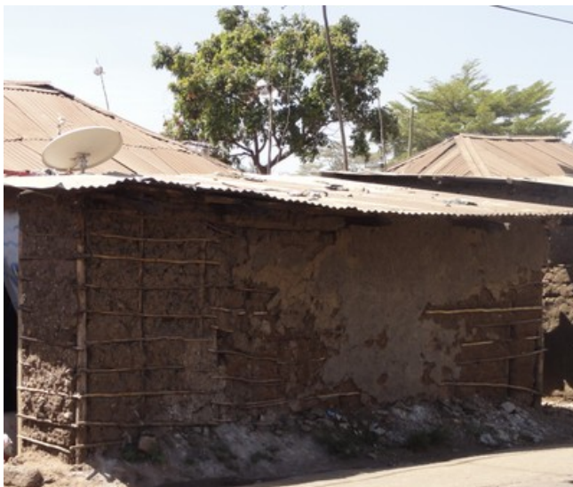
Mud walls reinforced with bamboo reinforcement, Kenya (K. Jaiswal)
