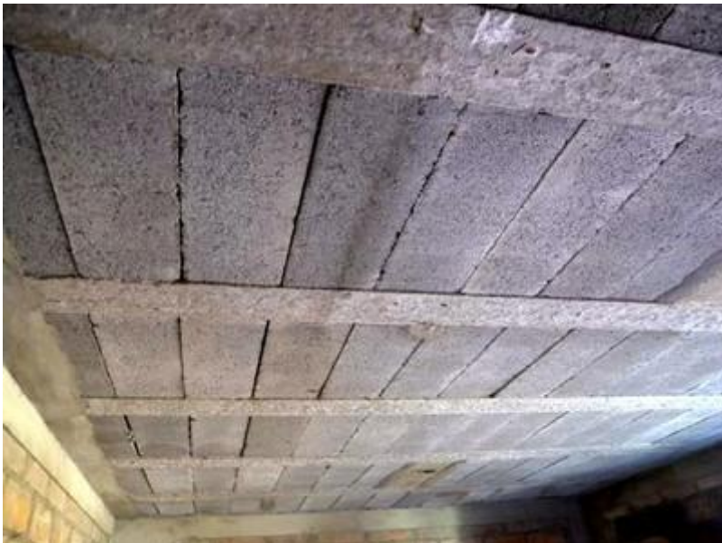
Roof/floor system consisting of concrete masonry units and cast-in-situ reinforced concrete joists (known as "Tralix" system), Chile (S. Brzev)
