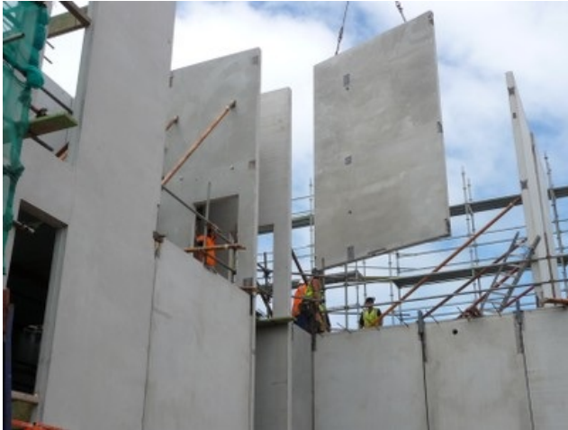
Erection of precast concrete wall panels, New Zealand (A. Charleson)
