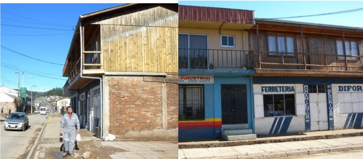
A building with a hybrid lateral load-resisting system consisting of the confined masonry construction at the first storey and timber construction at the second storey, Constitution, Chile (S. Brzev)
