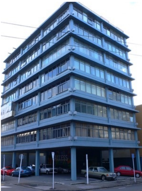
Soft storey in a reinforced concrete building, New Zealand (A. Charleson)
