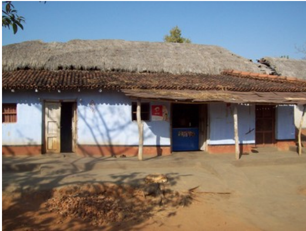
Cob construction, India (overlaid by plaster) (People in Centre)
