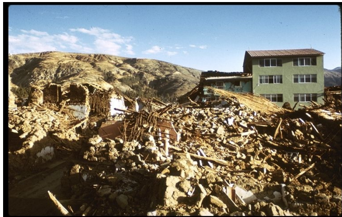
Photo 1 Destruction of adobe houses in Huaraz with 3-storey reinforced masonry building surviving the shaking
