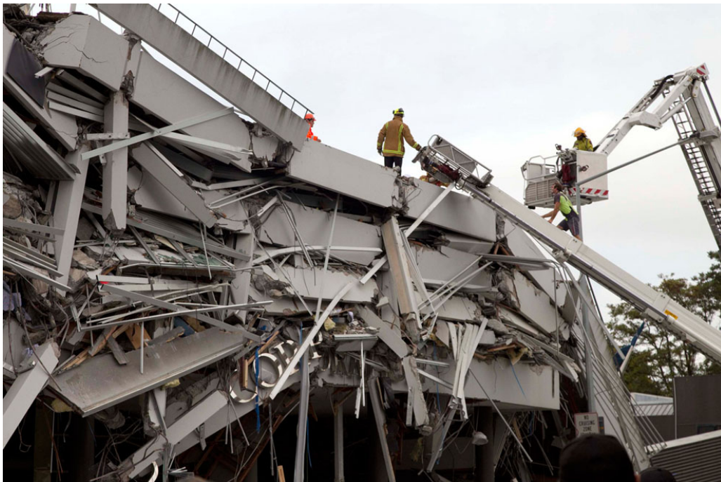
Photo 4 Catastrophic collapse of the Pyne Gould Corporation Building in the Central Business District of Christchurch, New Zealand
